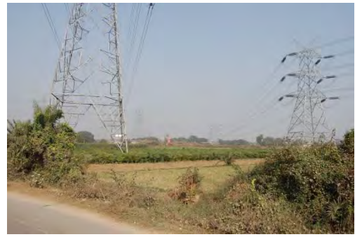
Existing Transmission line at Barh Taal area
