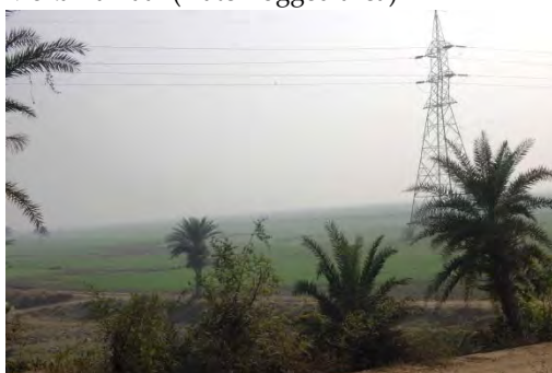
Existing Transmission Line in Mokama Taal area
