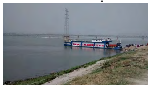
River Ganga and existing Transmission line
