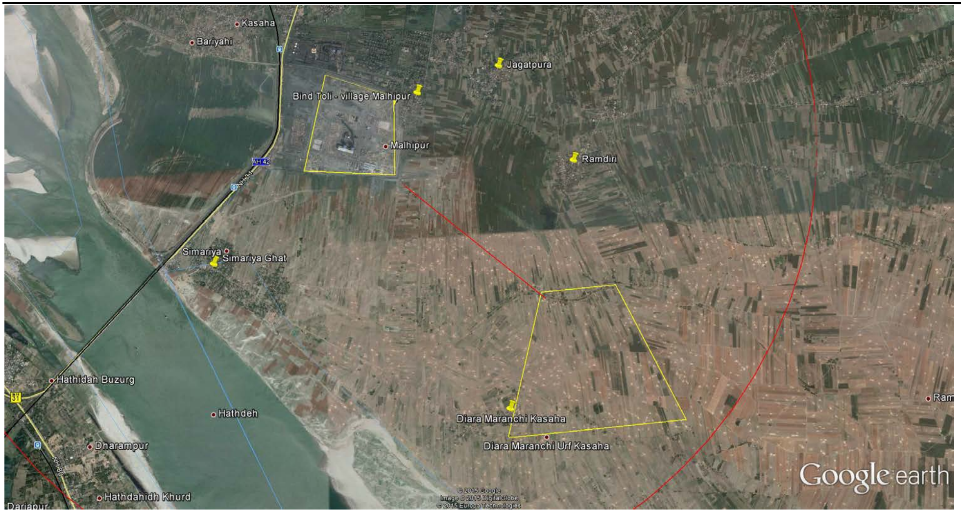
Figure 2.1 Main Plant Area and Project Components
