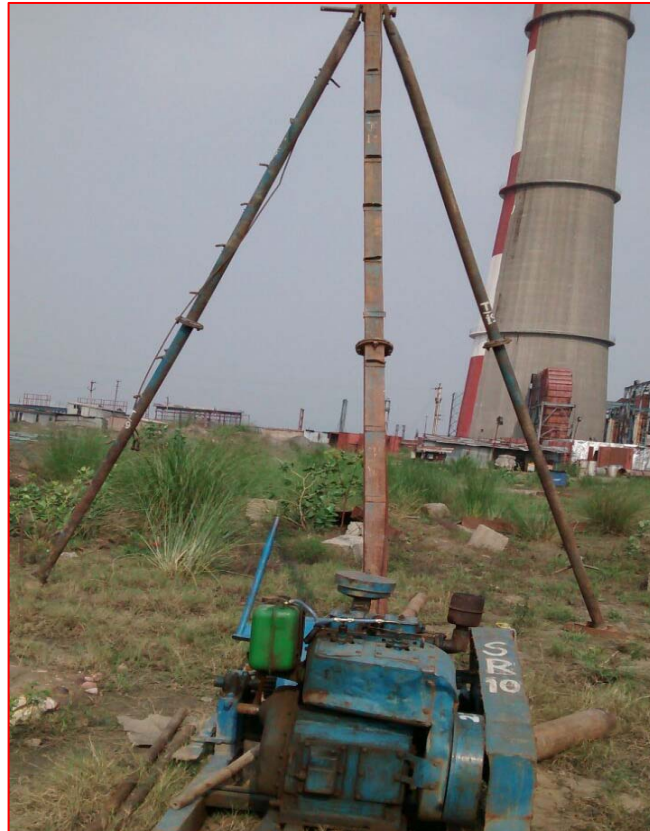
Photo: 3 Borehole No. BH-P3
