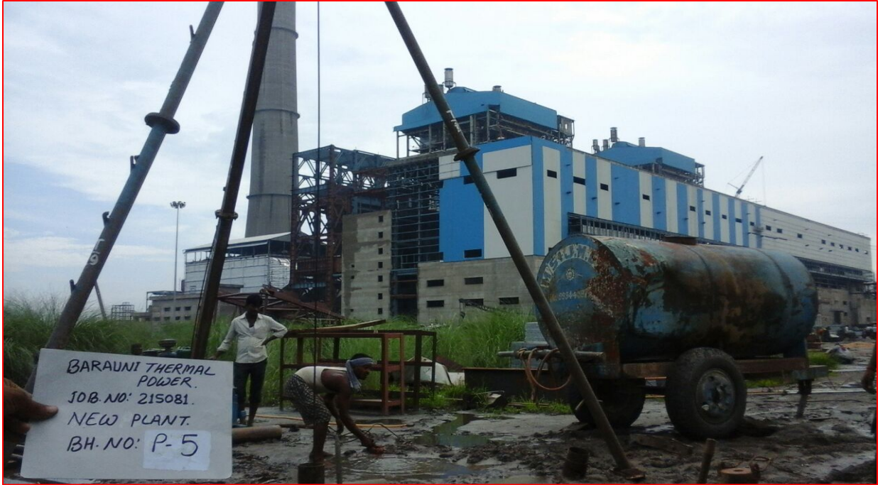
Photo: 5 Borehole No. BH-P5
