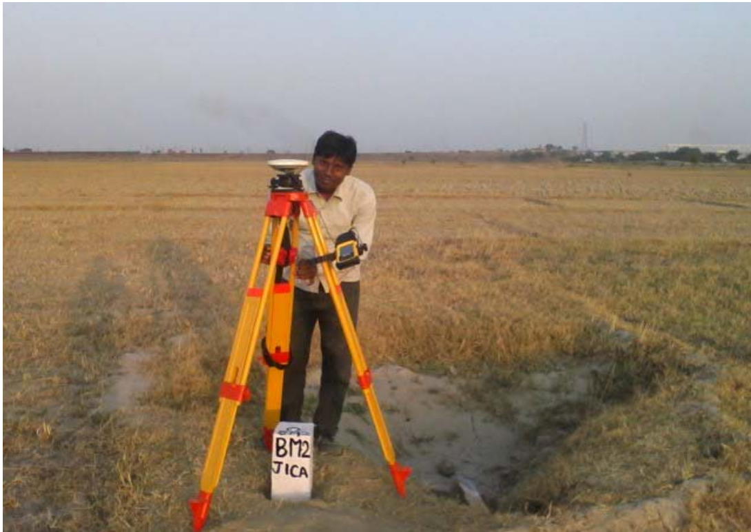
1. Photo no.1 shows DGPS Establishing a TBM.
