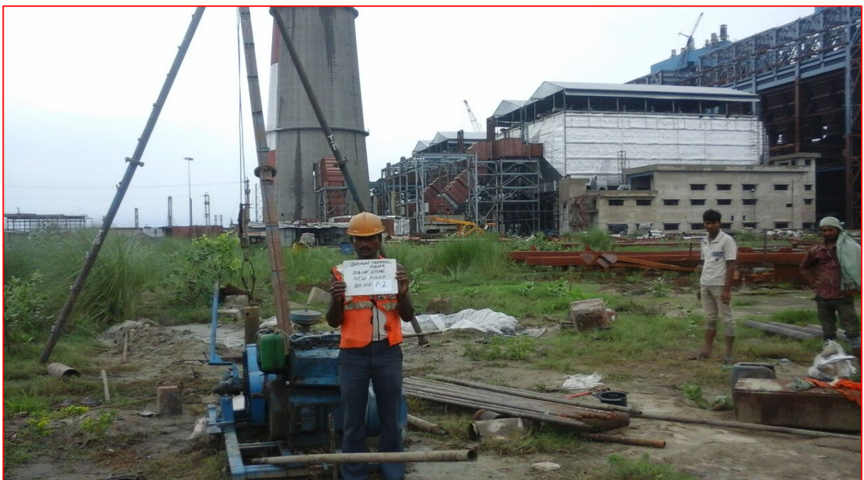
Photo: 2 Borehole No. BH-P2
