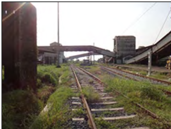
Railway Line Inside BTPS
