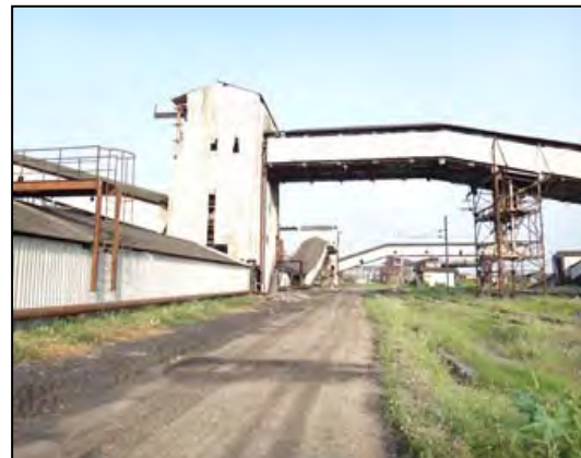
Conveyor & Transfer Point
