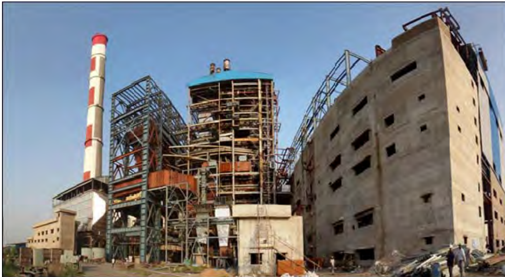
Figure 3.1-8 Construction of Unit No. 9 (Boiler-Turbine-Generator Area)
