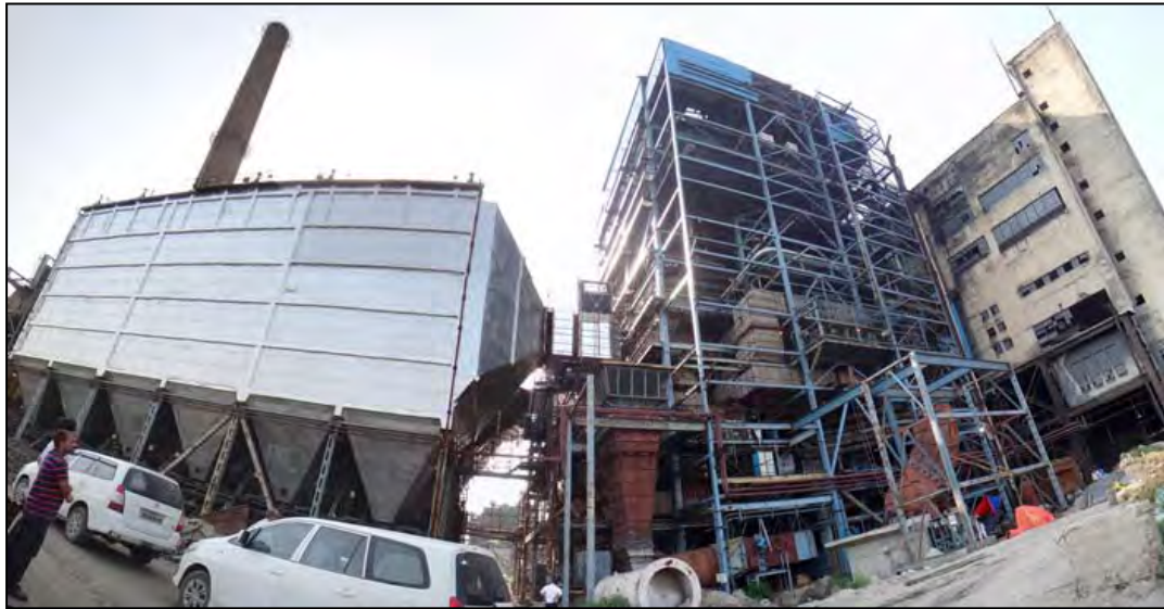
Figure 3.1-4 R&M/LE Status of Unit No. 7 (Boiler-Turbine-Generator Area)
