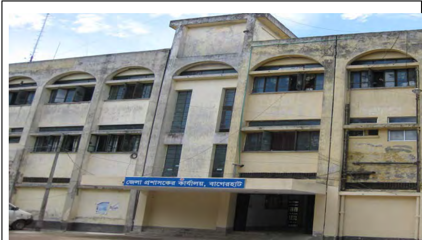
Photo-28 Bagerhat DC Office (DRR Office is the third floor.)
