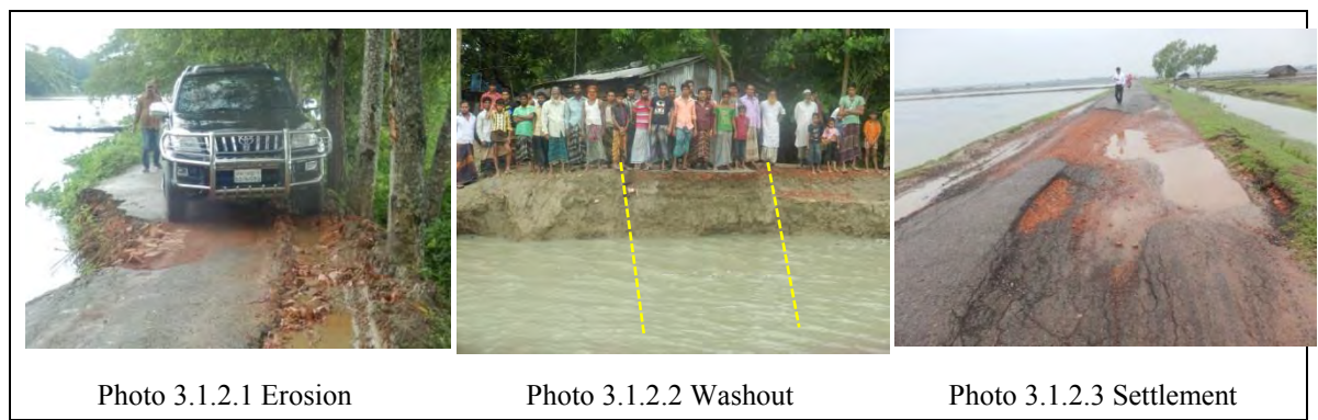
Figure 3.1.5 Photos of Damaged Roads
