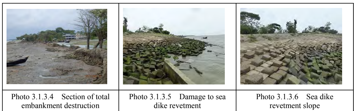
Figure 3.1.9 Photos of Damaged Coastal Dike
