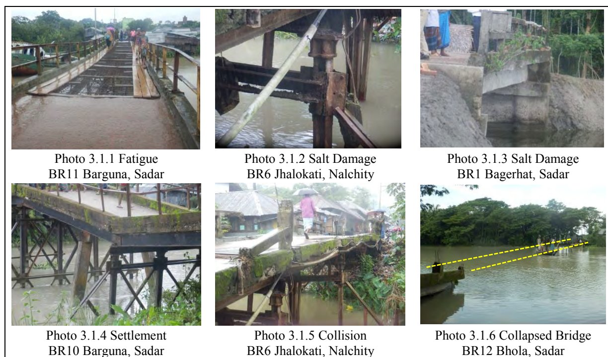
Figure 3.1.3 Photos of Damaged Bridges
