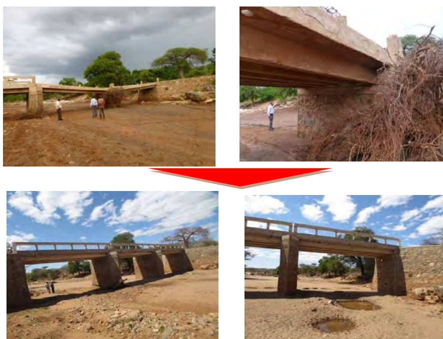
Figure2-21 Before and After the rehabilitation of bridge in Iringa DC
