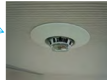
Sprinkler Head for false ceiling
