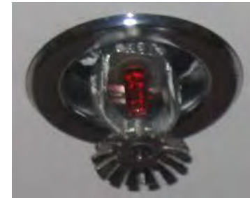
Sprinkler Head for Exposed
