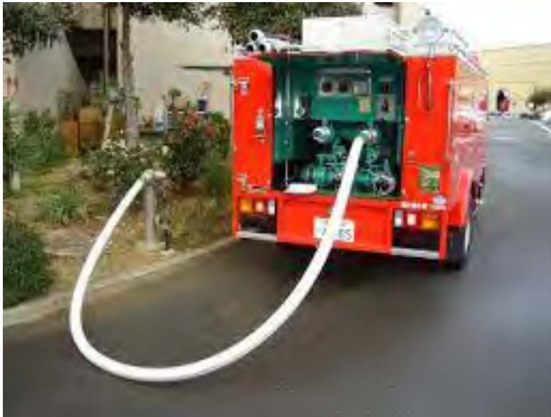
Fire Engine Supply water to Siamese Connection
