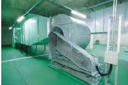
Centrifugal Fan for Tunnel Ventilation
