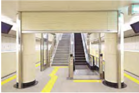
Smoke/Fire Protection Shutter
