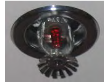
Sprinkler Head for Exposed
