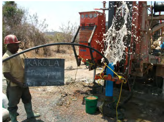
Figure 34 Development by Single-Tube Air-Lifting
