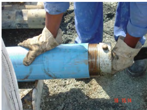
6. Fixing lifting cap on the lower end screen
