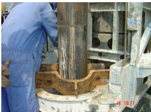
3. Fixing clamp on pulled out temporary casings
