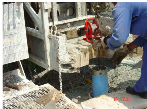
Figure 32 Measurement of Gravel Top
