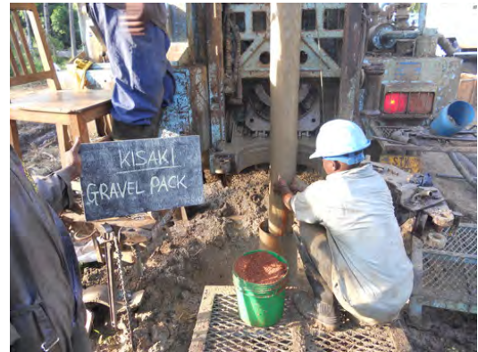
Figure 31 Installation of Gravel Pack
