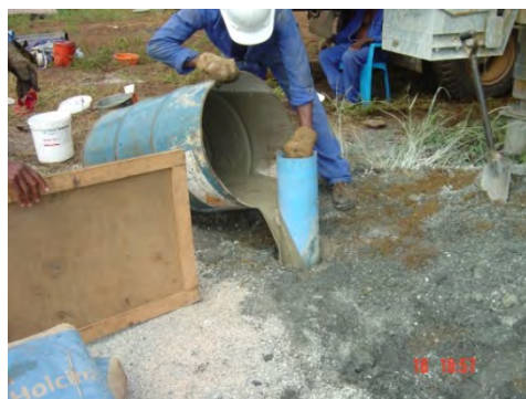
2. Slurry poured into the borehole
