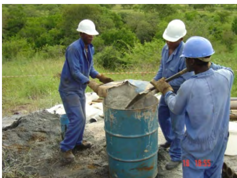
1. Mixing of cement slurry
