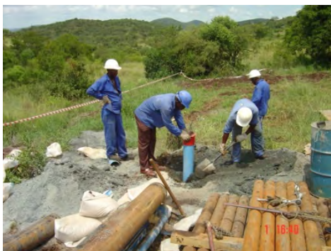
5. Well casing equipped with temporary well cap
