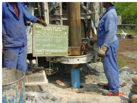
4. Removal of temporary casing from the well
