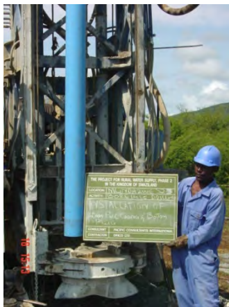
3. Installation of bottom plug & sump pipe
