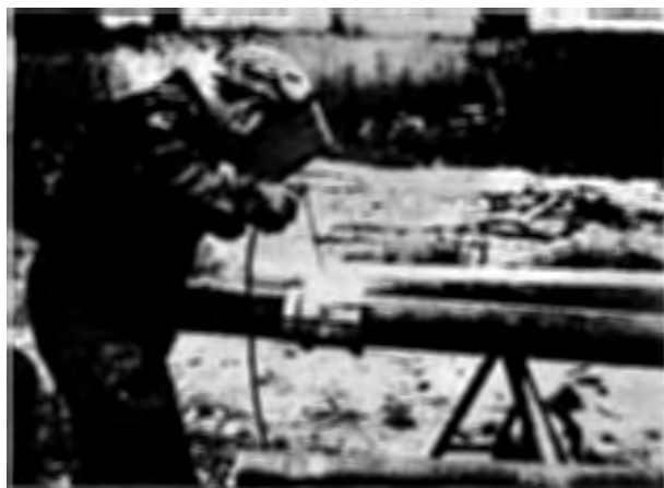
Fig. 45. Welding smooth casing tubes with the welding fixture Electric welding, employing a small, portable petrol-driven welding set as power aggregate, is much easier to perform than gas welding
