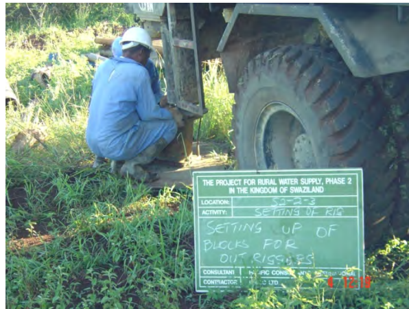
Figure 2 Fixing the jacks (out rigger) of the drilling rig
