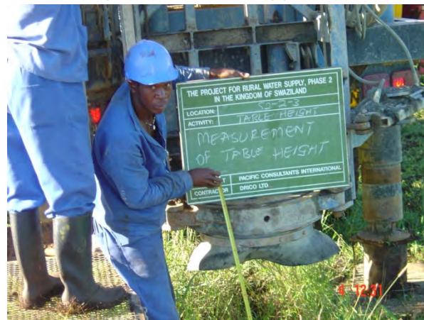
Figure 2 Fixing the jacks (out rigger) of the drilling rig
