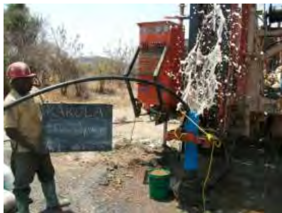
Figure 34 Development by Single-Tube Air-Lifting
