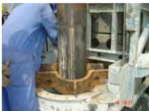
3. Fixing clamp on pulled out temporary casings
