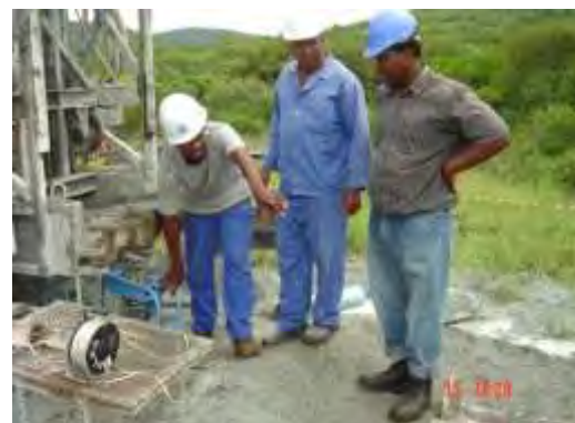
4. Explaining the installation of sheave stand on top of the borehole
