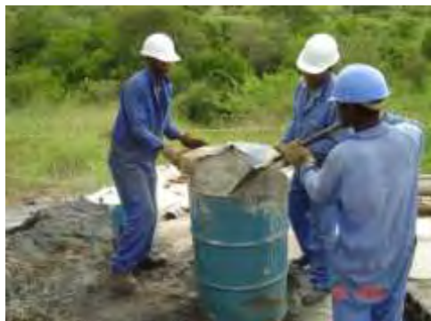
1. Mixing of cement slurry
