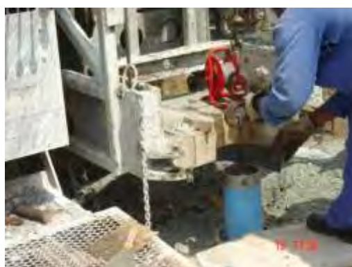
Figure 32 Measurement of Gravel Top
