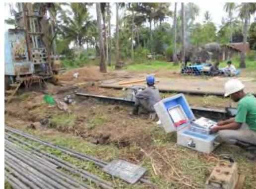
12. Carrying out the borehole logging
