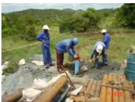
5. Well casing equipped with temporary well cap
