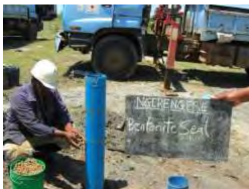
Figure 33 Installation of clay pellets
