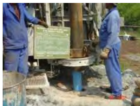
4. Removal of temporary casing from the well
