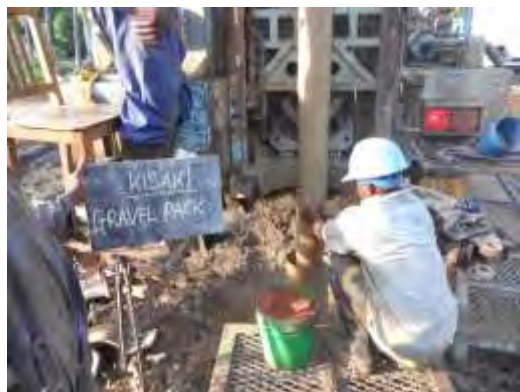
Figure 31 Installation of Gravel Pack
