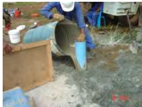
2. Slurry poured into the borehole
