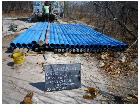
1. PVC well assembly according to the plan laid out on site
