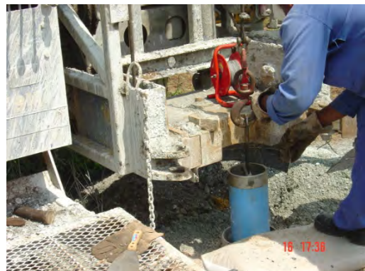
Figure 32 Measurement of Gravel Top
