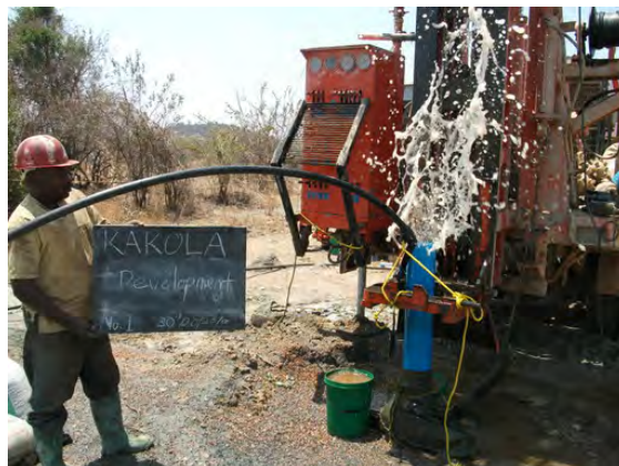
Figure 34 Development by Single-Tube Air-Lifting
