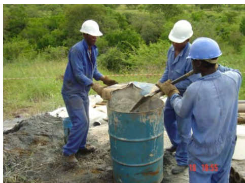
1. Mixing of cement slurry
