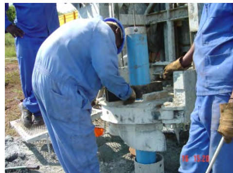
7. Fixing of camp to hold the pipes on the working place
