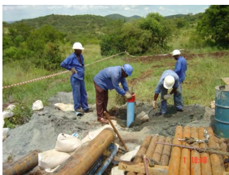
5. Well casing equipped with temporary well cap
