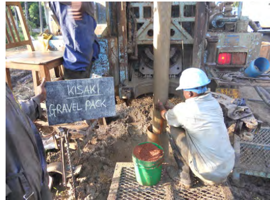
Figure 31 Installation of Gravel Pack
