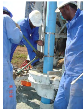
5. Cutting bolts of centralizer
