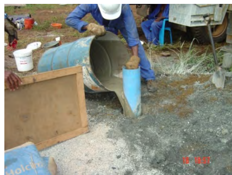
2. Slurry poured into the borehole
