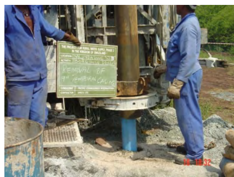
4. Removal of temporary casing from the well
