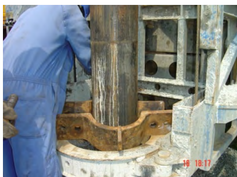
3. Fixing clamp on pulled out temporary casings
