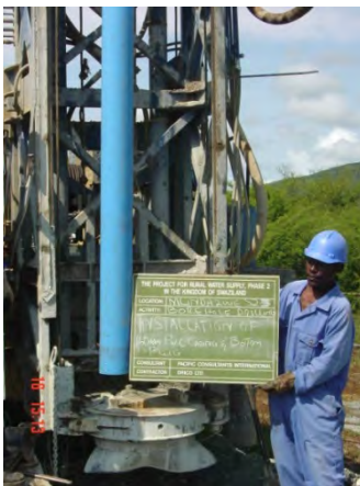
3. Installation of bottom plug & sump pipe
