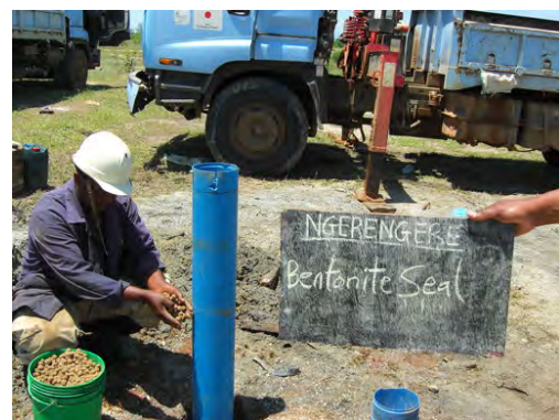
Figure 33 Installation of clay pellets
