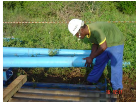
2. Cutting bolts of centralizer
