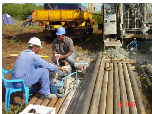
13. Trainee personnel running the borehole-logging
