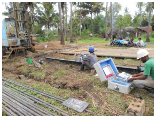
12. Carrying out the borehole logging
