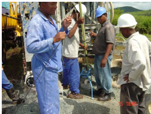
10. Inserting the probe into borehole
