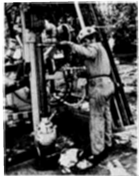
Fig. 13b. Put the breaking wrench in the wrench recess and apply force by hand turning to the left
