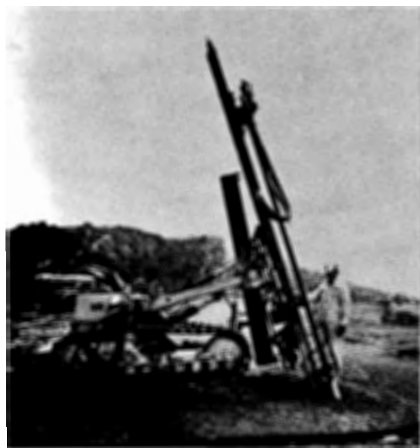
Fig. 8. By loading the feed spike with a portion of the weight of the wagon drill a solid set-up can be obtained (ROC 301 with COP 4)
