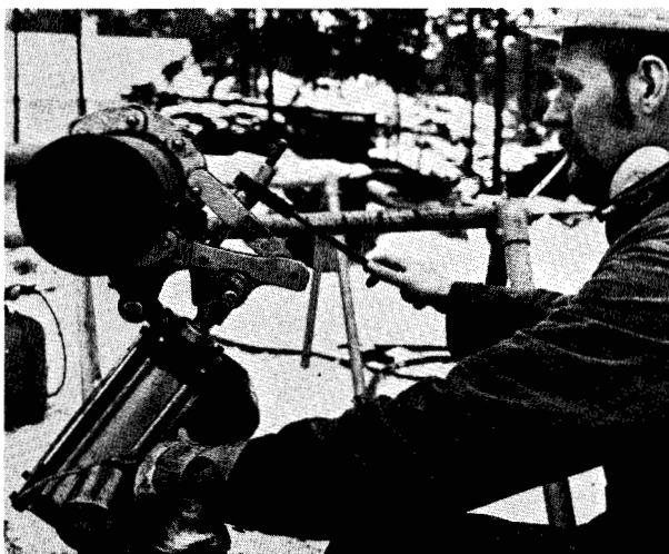
Fig. 42. Semi-automatic, pneumatic tube cutter ensuring a perfect 90° cut, a prerequisite for easy and safe welding
