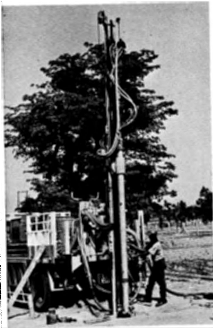
Fig. 38. Water well drilling through soil with Aquadrill 461, incl. feed BMM 36K 855, rotation unit BBR 6 and down-the-hole drill COP 4
