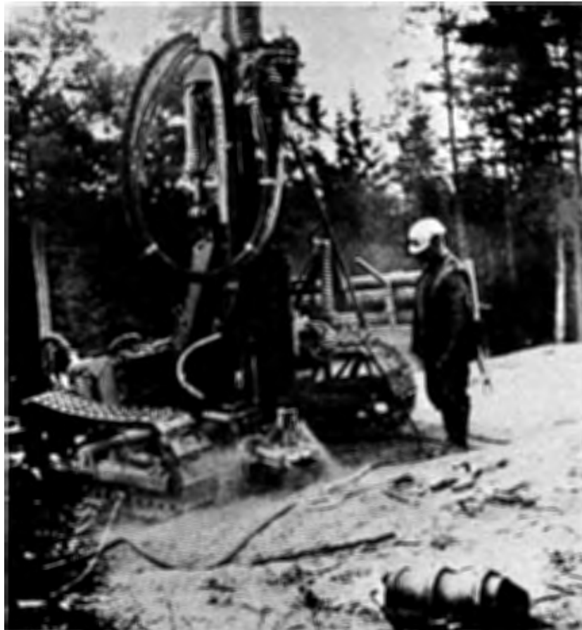
Fig. 27. Metering the liquid foaming mixture into the compressed air
