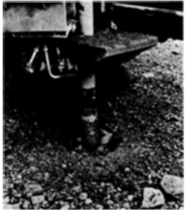
Fig. 24. An unstable surface layer collapses easily and may make drilling impossible
