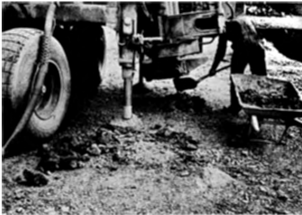
Fig. 25. Filling the upper part of the drill hole with clay
