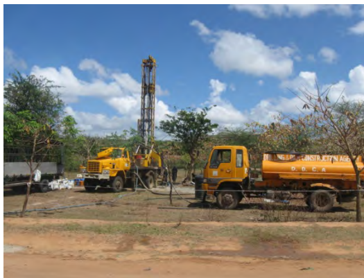
Source: JICA's Rural Water Supply Project in Metropolitan Area in Tanzania
