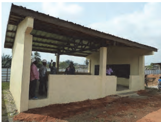
South East Side View
