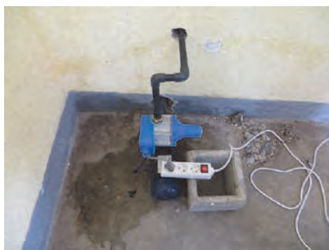
Insulation of Booster Pump in GS SOGEFIHA 6
