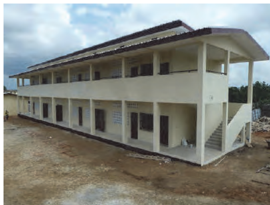
Completion of Work (June 2015)
