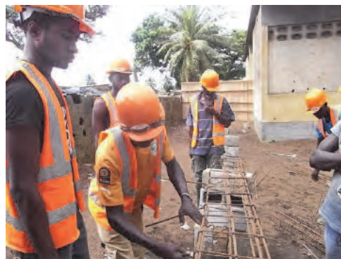
Trainees learning Iron work (Yopougon)
