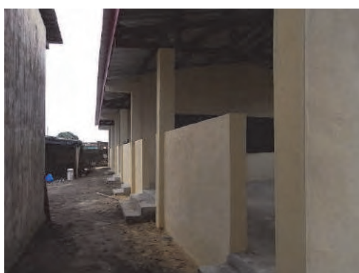
Entrance of Classroom
