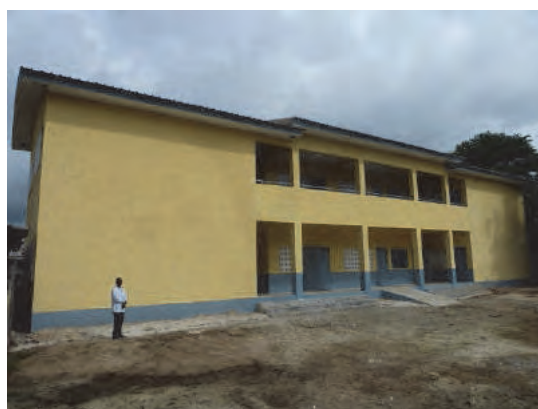
Completion of Work (June 2015)
