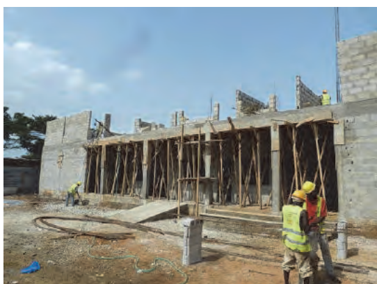
External Wall (March 2015)
