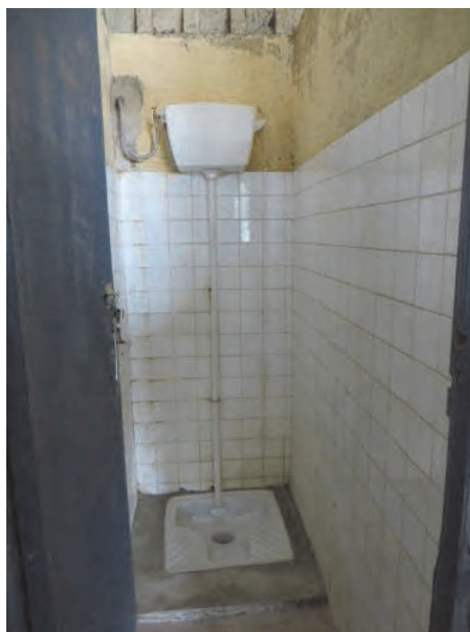
Sanitary facilities of GS Palmeraie
