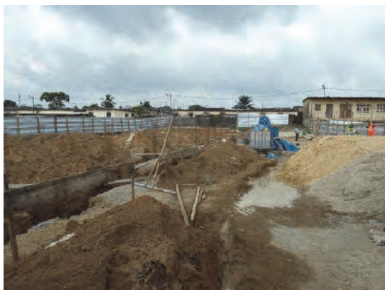
Foundation Work (January 2015)
