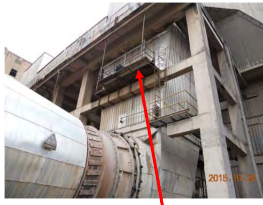
Photo 4-4b Measurement point at outlet of ESP
