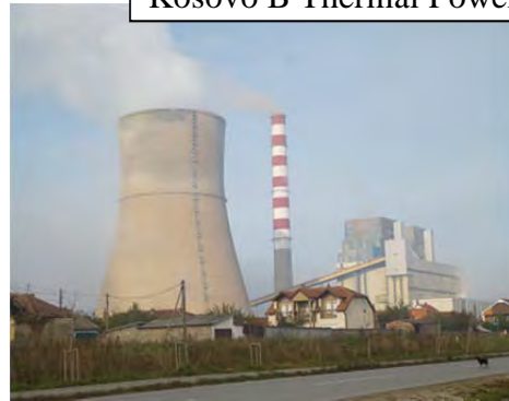
Kosovo B Thermal Power Plant
