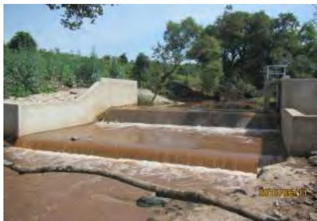
Completed Intake Weir
