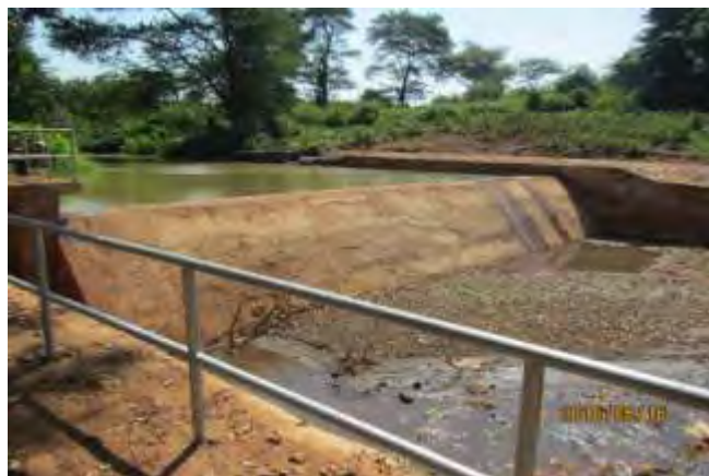
Intake Weir after Rehabilitation Works
