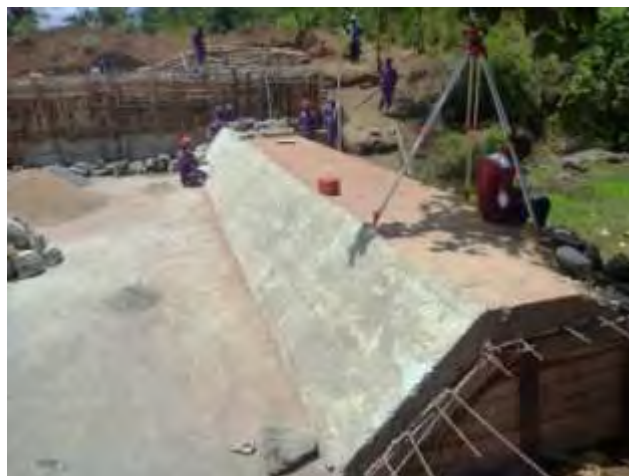
Intake weir under Construction
