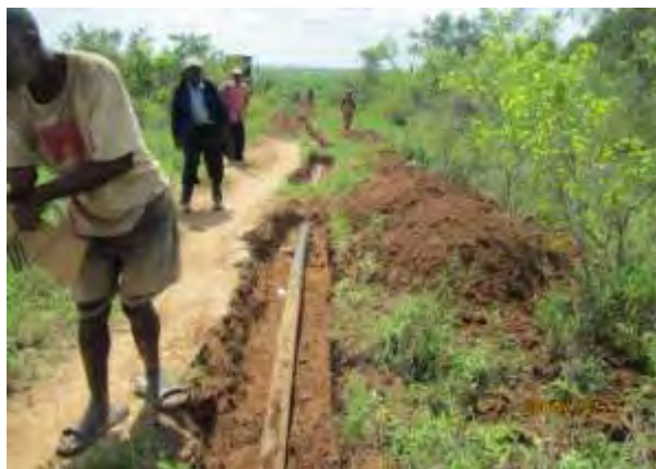
Pipe Laying Works
