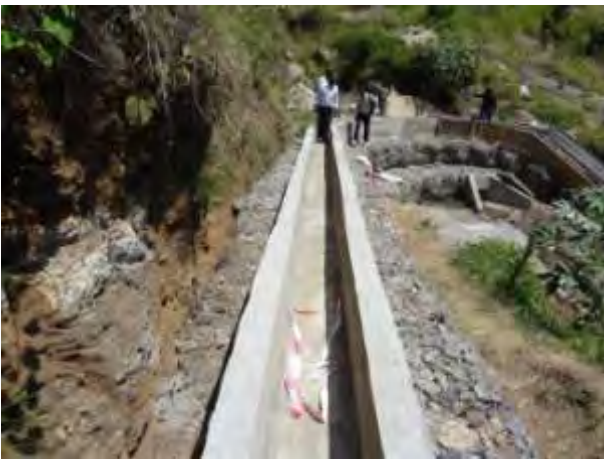
Canal Lining Works
