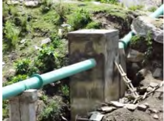
Construction of Stream Crossing
