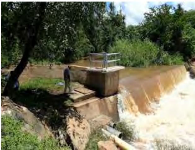
Rehabilitated Intake weir
