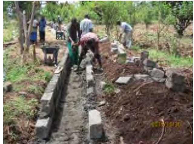
Canal Lining Works
