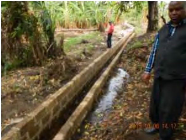
Canal Lining Works by IWUA members
