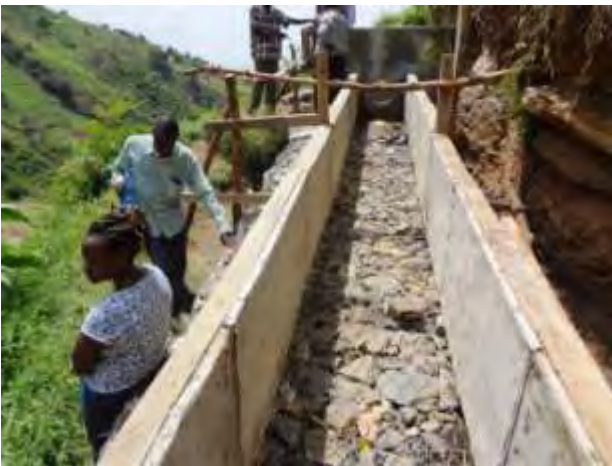
Construction of Stream Crossing
