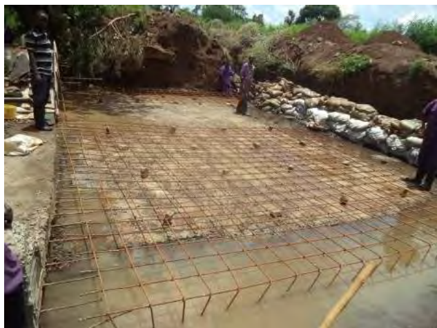
Intake Weir under Construction
