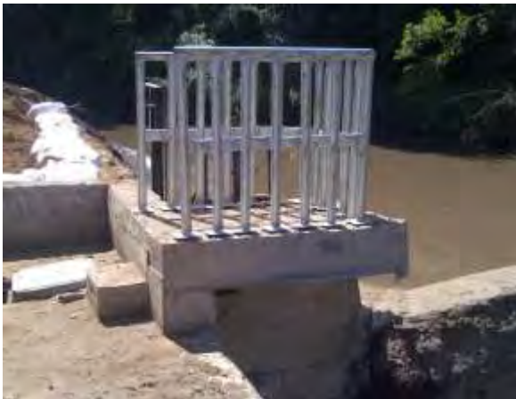
Rehabilitated Intake Weir
