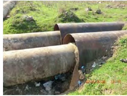
Figure 3.2.1-5 Pipeline of hot water supply (on the right: aboveground part; on the left: underground part)
