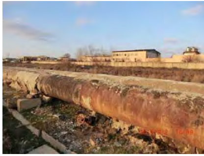
Figure 3.2.1-5 Pipeline of hot water supply (on the right: aboveground part; on the left: underground part)
