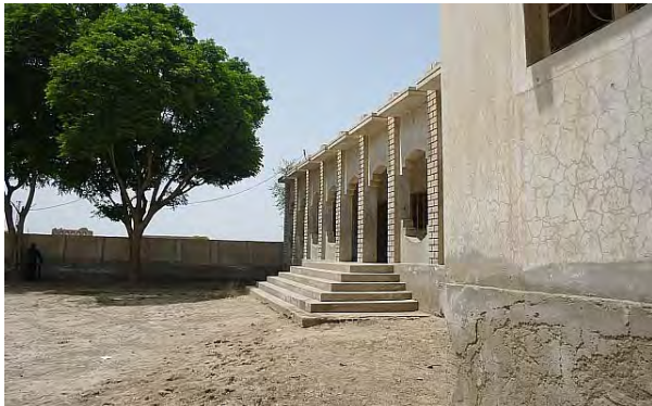
Da01 GGPS Kamaluddin Village Kanhiri: 既存校舎外観。
