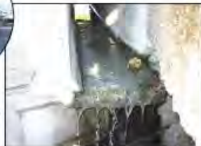
A road gully in tandoku-johaksou installation area in 1970s, (where whitish sludge was attached to)
