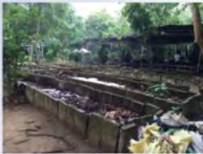
Composting site in Kaluna-san: Lack of access road for truck -> Unusable
