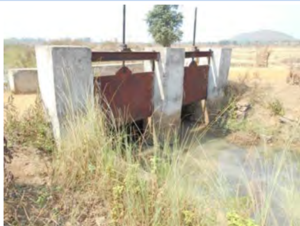
Right Main Canal: Regulator and Bridge
