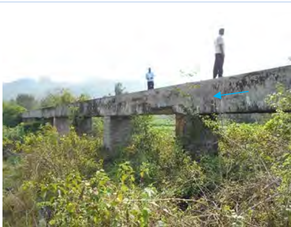
(Right Main Canal) Aqueduct: Reconstruction
