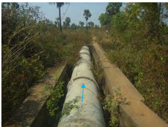
(Left main canal) Aqueduct: Reconstruction
