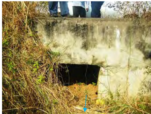
Right Main Canal: Distributor_UT (Drain Syphon)
