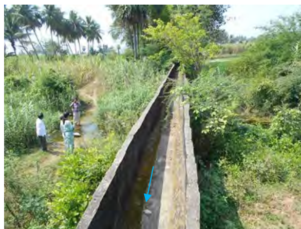
(Left Main Canal) Aqueduct: Reconstruction
