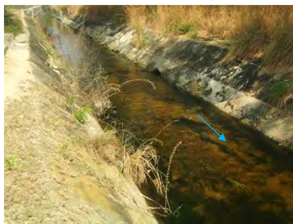
(Left Main Canal) Concrete Lining: Reconstruction
