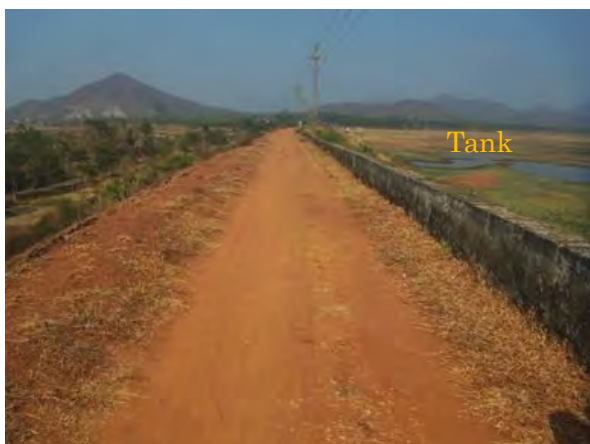
(Dam) Top of Bund (Dam): Repair
