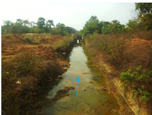
(Left Main canal) Wall type canal: Reconstruction
