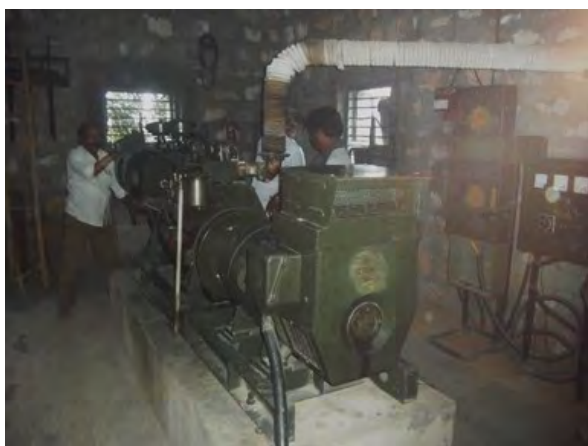
(Generator House) Generator: Replacement
