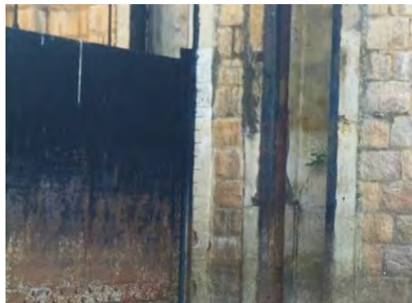
(Spillway) Rubber seals of gates: Replacement
