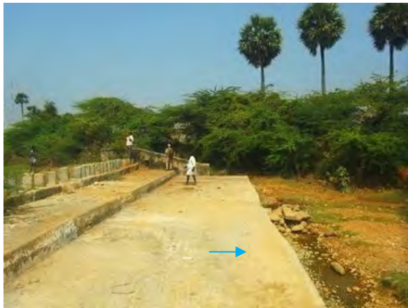
Surplus Weir : Reconstruction
