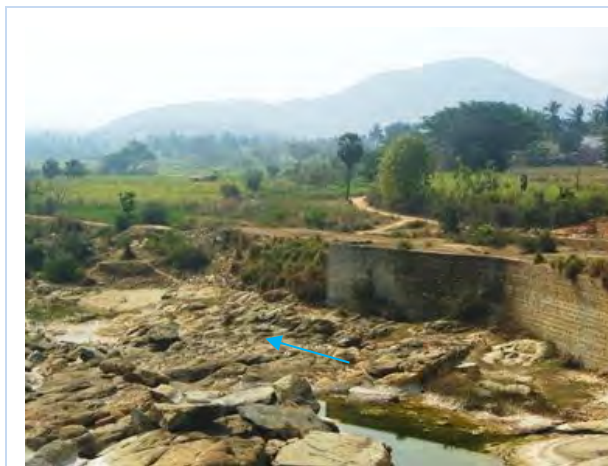
(Spillway) Eplon: Repair
