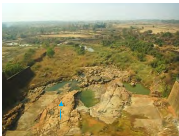
(Spillway) D/S apron: Repair
