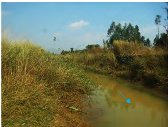
Right Main Canal: Lining
