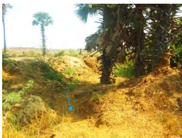
Feeder canal : Reconstruction
