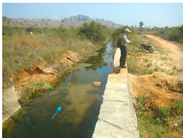
(Left Main Canal) Off take 1: Reconstruction
