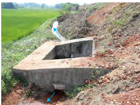
Supply Channel 1 : Reconstruction
