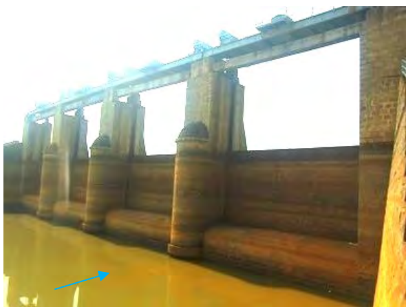
(Spillway) Gates: Replacement (wire ropes, rubber seals, painting etc.)
