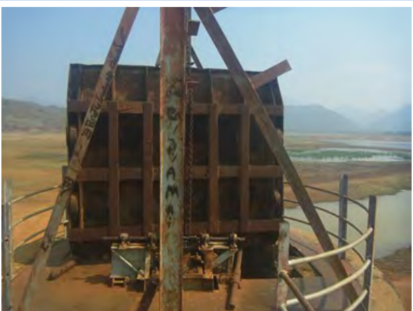
Intake of Left Side: Replacement (concrete and sluice gate)
