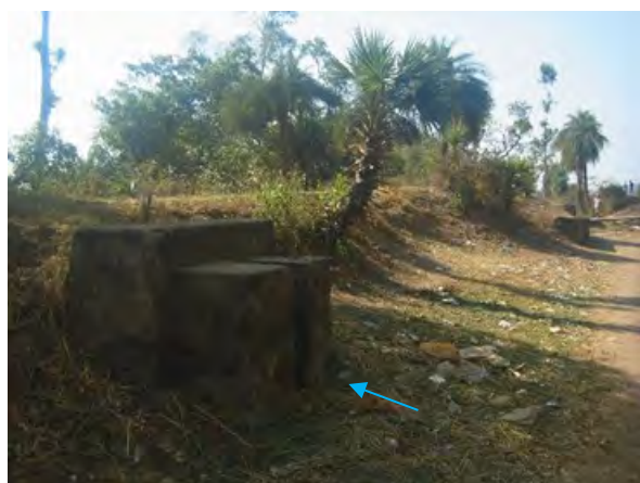
Drain Channel (downstream of the surplus weir) : Reconstruction
