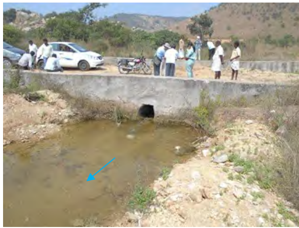
(Left Main Canal) Off take 1: Reconstruction
