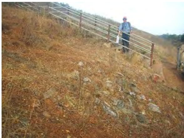
(Dam) Toe drain: Repair
