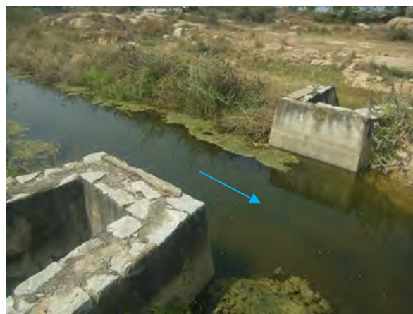
(Left Main Canal) Under Tunnel (Syphon): Reconstruction
