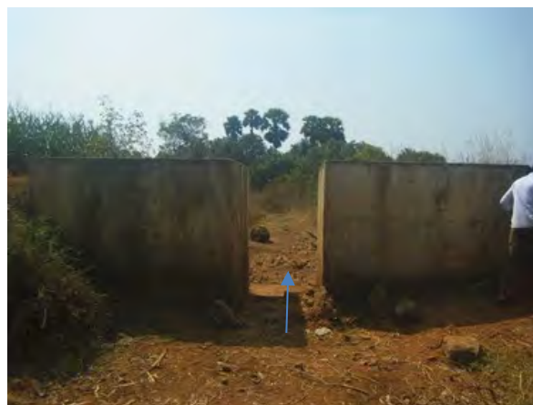
(Left main canal) Regulator: Replacement of gate
