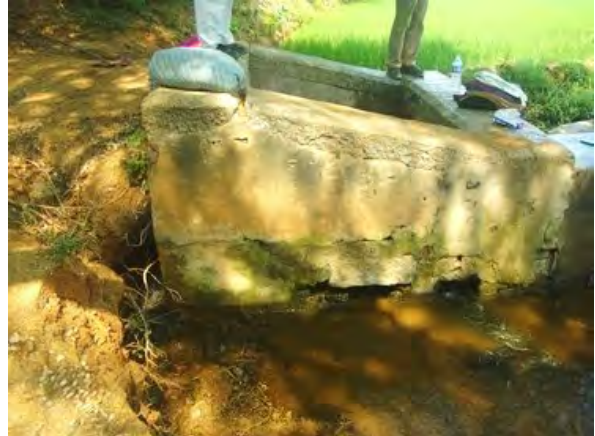
Supply Channel 2 : Reconstruction
