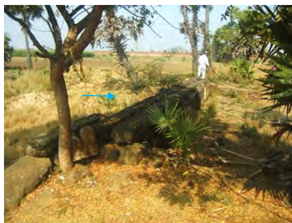
Surplus Weir 1 : Reconstruction
