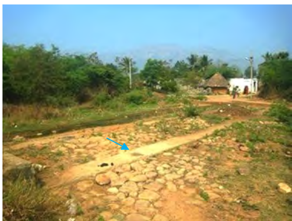
Surplus Weir : Reconstruction
