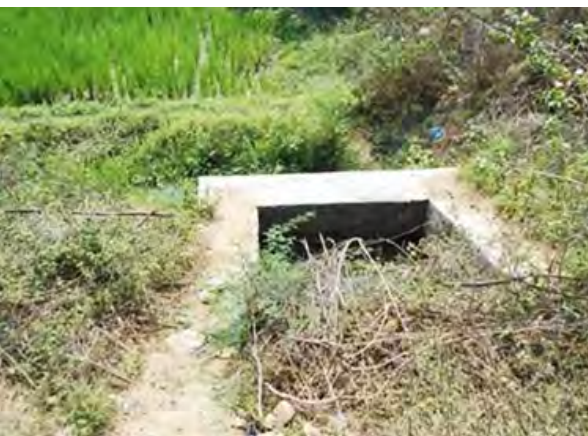
Supply Channel 1 : Reconstruction
