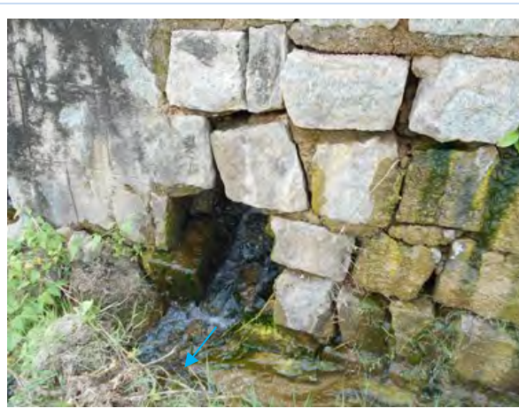
(Right Main Canal) Aqueduct: Reconstruction
