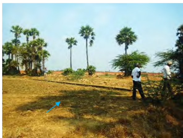
Surplus Weir 2 : Reconstruction
