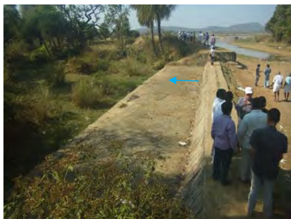
Surplus weir : Reconstruction
