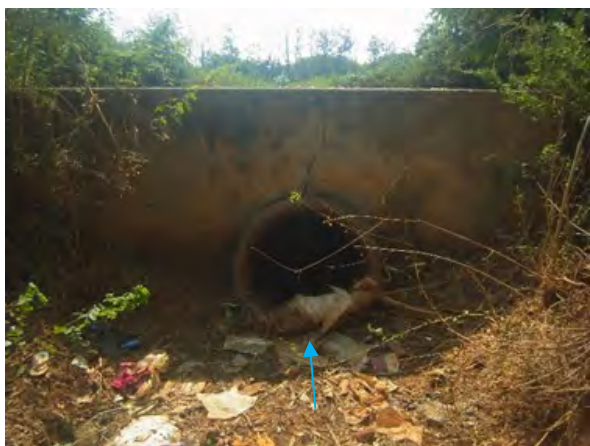
(Left main canal) Siphon: Reconstruction
