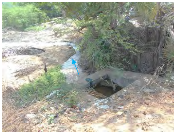
Supply canal 2 : Reconstruction
