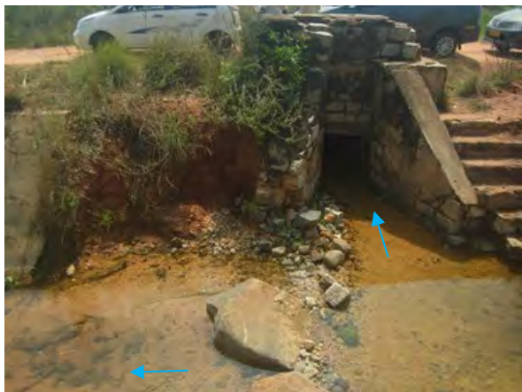
(Left Main Canal) Off take 2: Reconstruction
