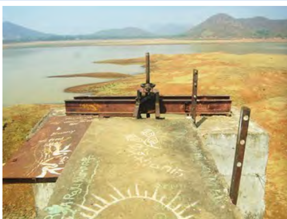
Intake of Right Side: Repair (concrete) and replacement (sluice gate)
