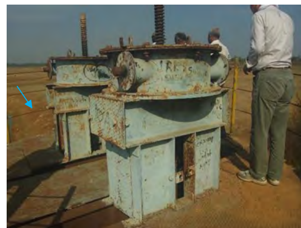
(Left side intake) Gate: Replacement
