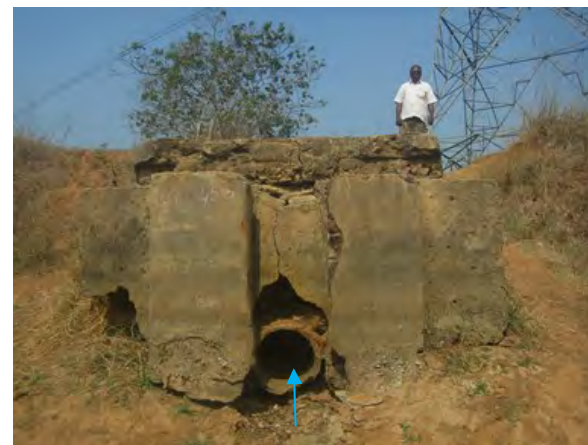
(Left main canal) Off take: Reconstruction
