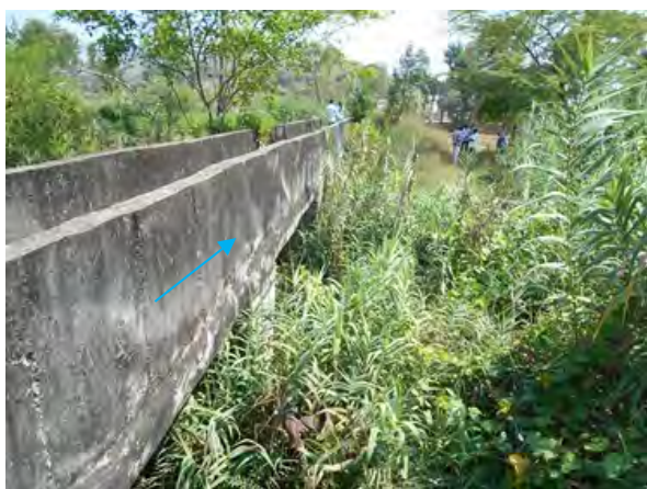
(Left Main Canal) Aqueduct: Reconstruction
