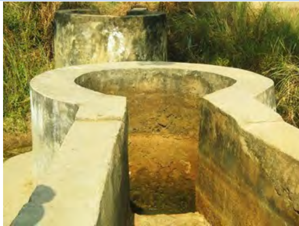
Right Main Canal: Distributor_Syphon
