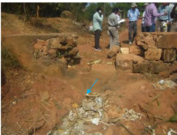
(Left main canal) Drop: Reconstruction
