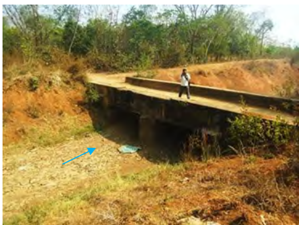
Right Main Canal: Distributor_Bridge
