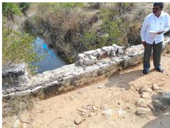
(Left Main Canal) Super Passage: Reconstruction
