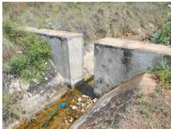
(Left Main Canal) Drop: Reconstruction
