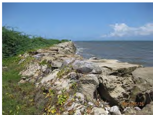
Photo Revetment nearby RWY 07
