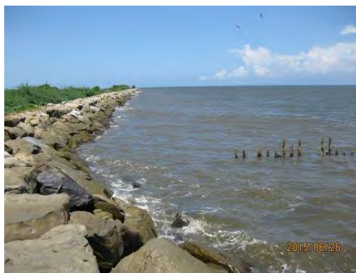
Photo Revetment nearby RWY 07
