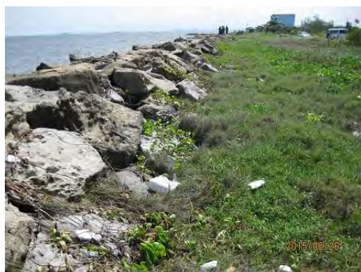
Photo Revetment nearby RWY 07
