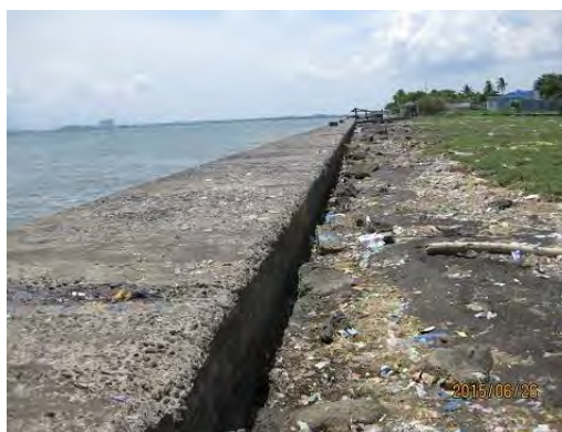
Photo Revetment nearby RWY 25 End
