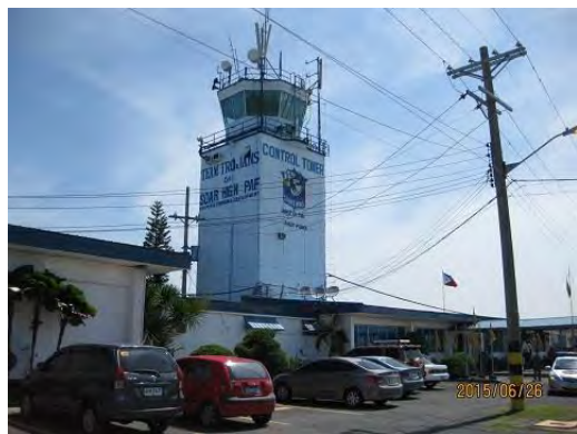
Photo Control Tower from Landside
