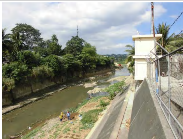
Elevated Nangka Station (January 2016)
