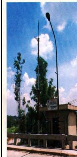
STO. NIÑO WATERLEVEL GAUGING STATION. Water-level gauging stations measure real time water elevations. This particular waterlevel gauging station is a major control point and is located on the left side of the Marikina Bridge along the upper Marikina River in Sto. Niño, Marikina.
