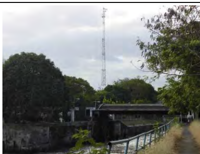
Newly constructed Tower at Napindan HCS (Feb. 2016)
