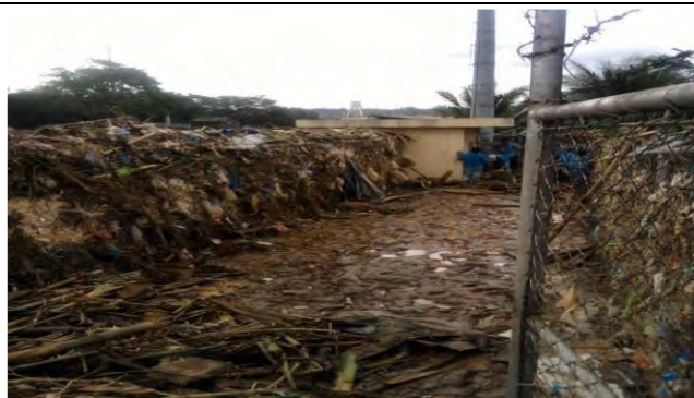
Nangka Observation Station damaged by flood caused by Typhoon Ondoy (photo by EFCOS Office) (September 2009)
