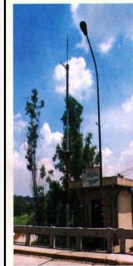
STO. NIÑO WATERLEVEL GAUGING STATION. Water-level gauging stations measure real time water elevations. This particular waterlevel gauging station is a major control point and is located on the left side of the Marikina Bridge along the upper Marikina River in Sto. Niño, Marikina.
