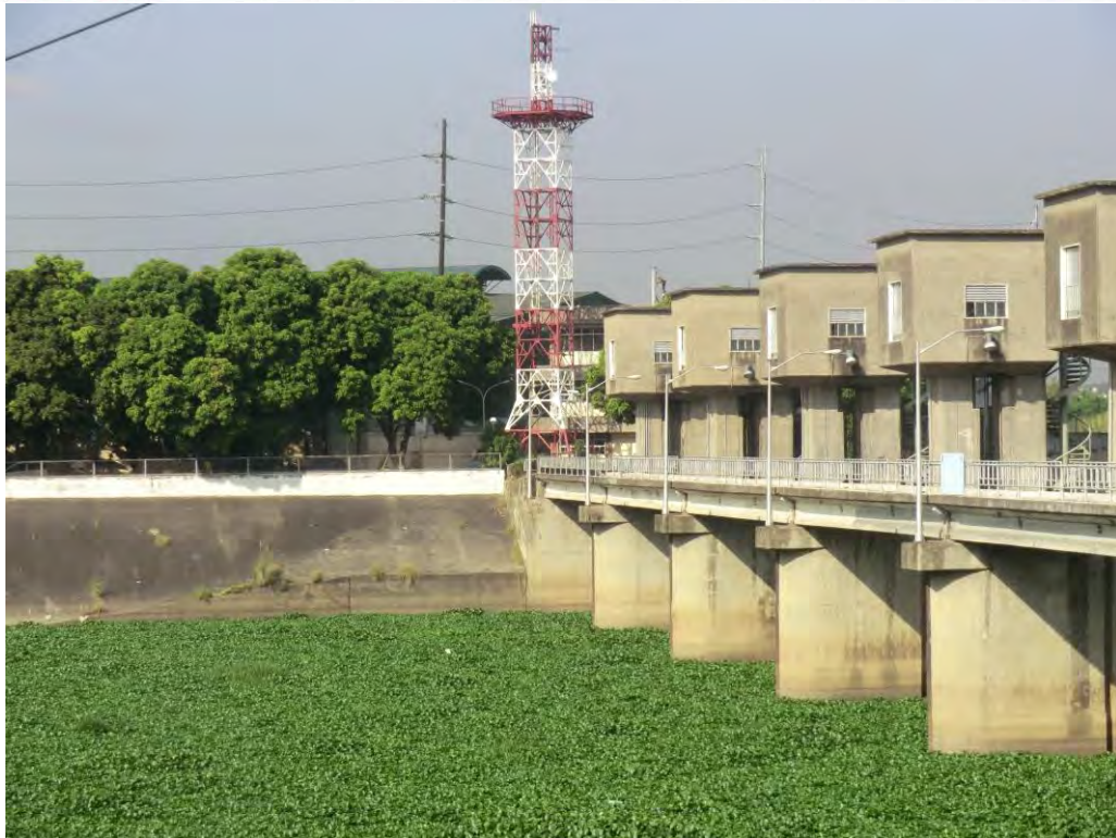
EFCOS Rosario Master Control Station and Rosario Well
