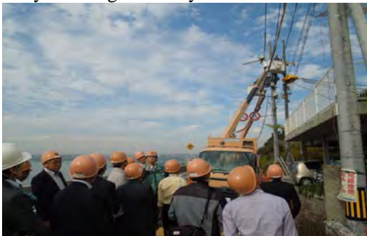
Job site inspection of Hot Line work
