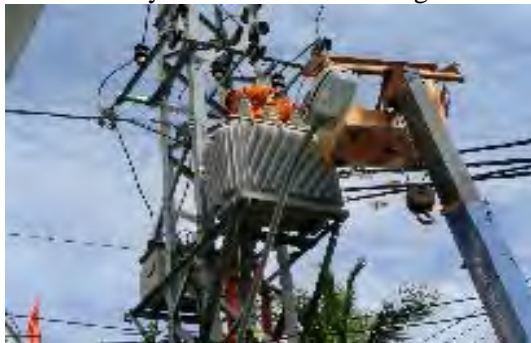
Hot Line work with US aerial work platform in Ho Chi Minh
