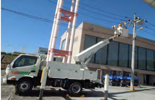
Aerial work platform for Hot Line work
