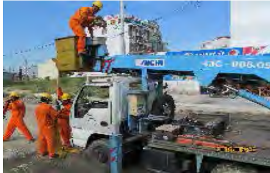
Aerial work platform for Off Line work in Da Nang
