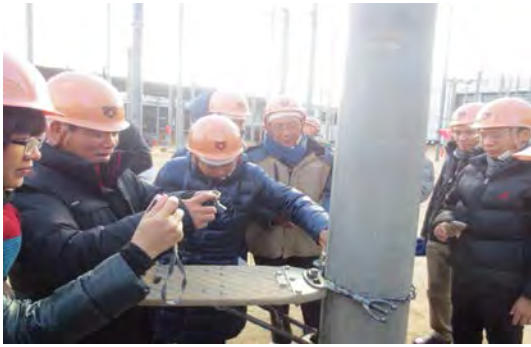
Demonstration of pole platform
