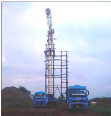
Photo 2-4.1 Power plant construction area
