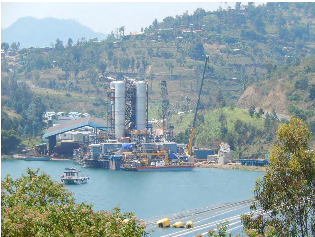
Photo 2-4.6 Methane extraction plant assembly site
