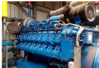
Photo 2-4.4 Engine for methane gas power generation
