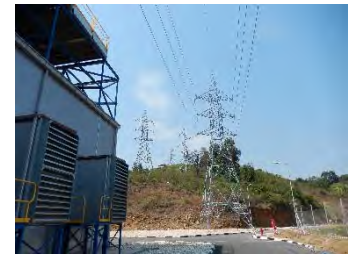
Photo 2-4.9 New installed transmission line for KivuWatt PS (11kV)
