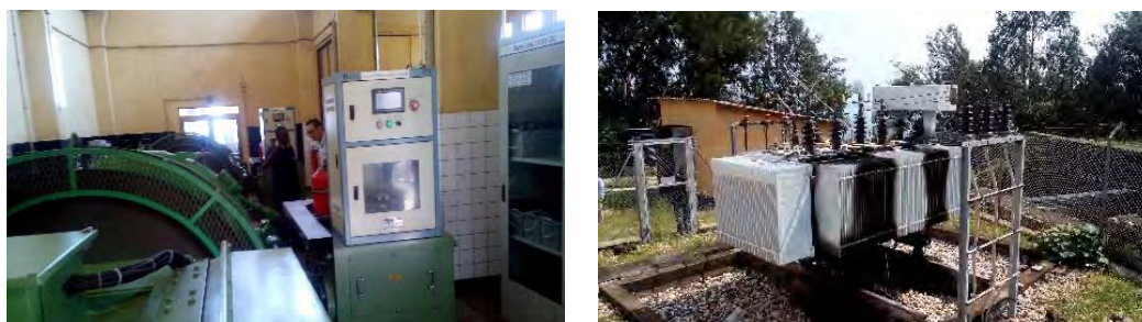
Photo 2-2.1 Gisenyi Power Station generator and transformer (insulating oil seemed to be leaking)
