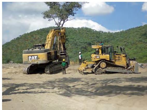
4 : Heavy machines; excavator and dozer
