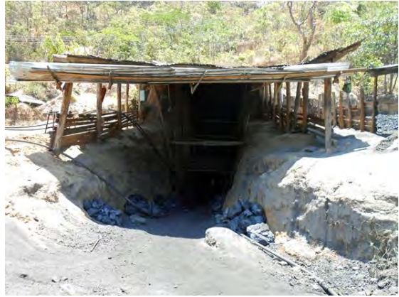
2 : Inlet of gallery for transport
