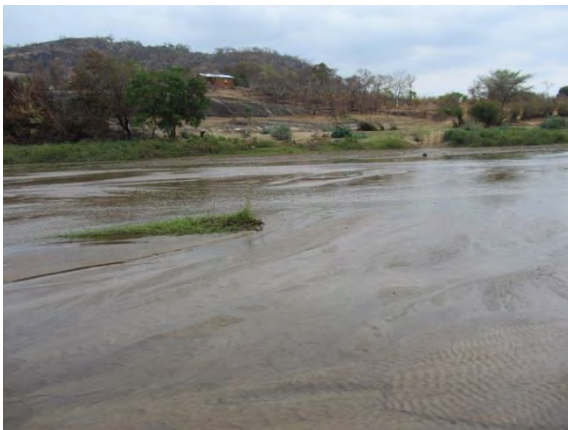
5: Road crossing river after unseasonal rain (Mzimba area)
