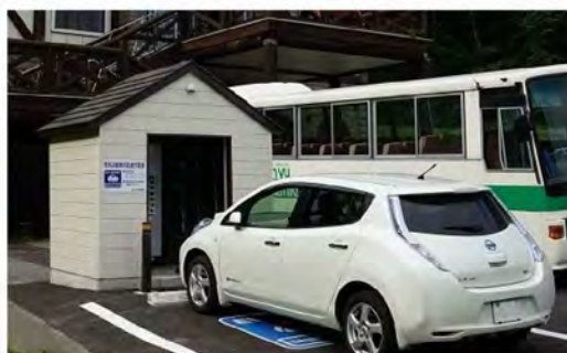
Indoor type Safety measure
