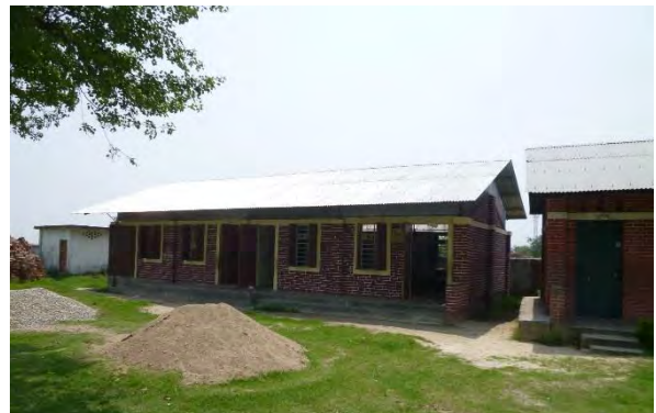
コミ開無償型: Shree Himali Primary school (JICA Grant Aid for Community Empowerment "Terai type")
