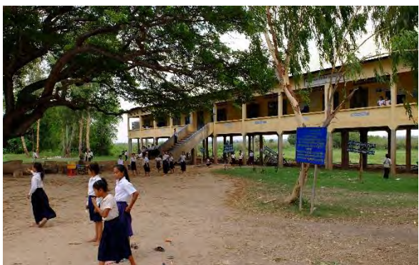
ADB 財政支援型: Tone Krao Primary School (Lower Secondary School 増築 by ESDPIII)
