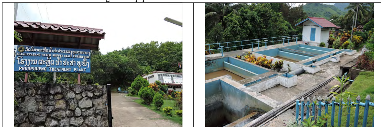
Figure 4.2.1 Phou Phueng WTP
