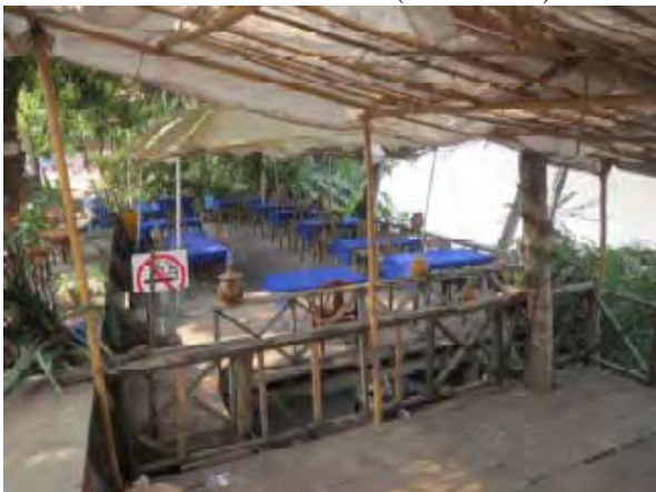
Terrace Deck (Not Allowed)
