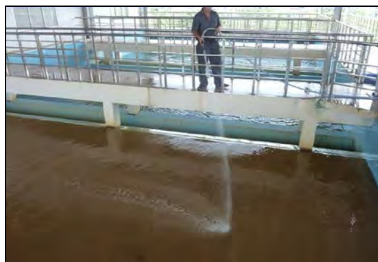
Photo 3.5 Rapid filtration Pond Workers spray water to remove scum on a regular basis
