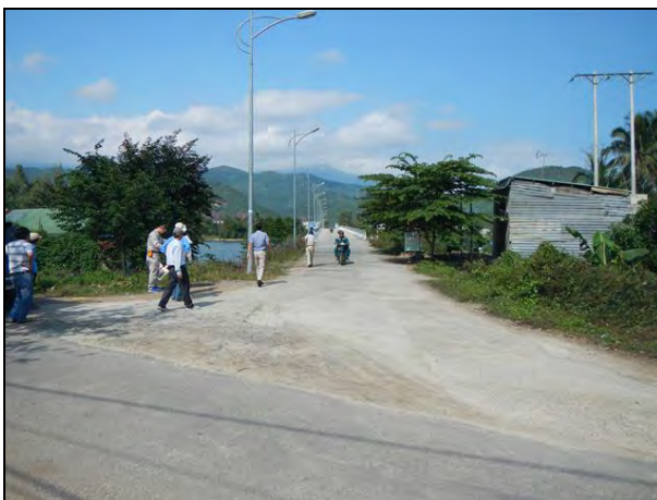
Photo 5.23 Trung Dinh bridge crossing Cu De river in Section h-i. Pipe lies left to right
