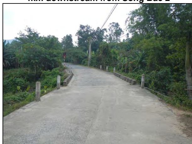
Photo 5.17 Typical view of road, Section a-b
