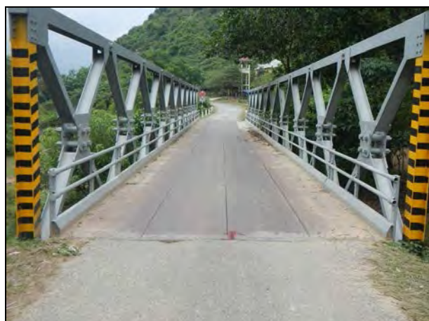
Photo 5.15 Existing Girder bridge at Nam My, 4km downstream from Song Bac 2
