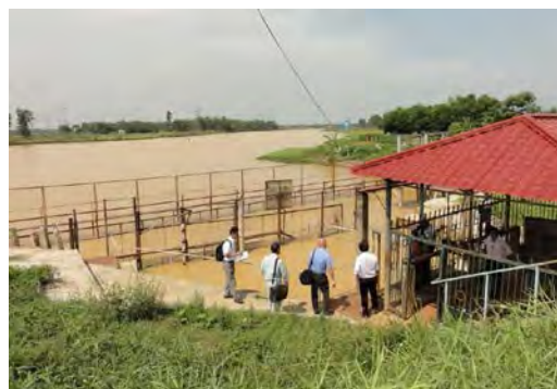
Photo 3.3 An Trach Weir constructed upstream of Cau Do River (Left photo taken in September 2013) and water intake point at Cau Do WTP (Right photo taken in June 2013) High level of turbidity can easily be identified.
