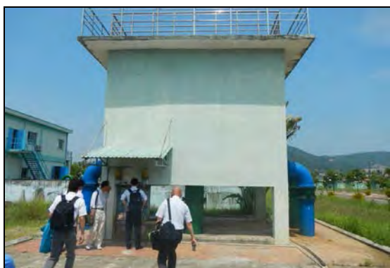
Photo 3.4 Receiving well in San Bay WTP Raw water is delivered from the receiving well in Cau Do WTP to this WTP
