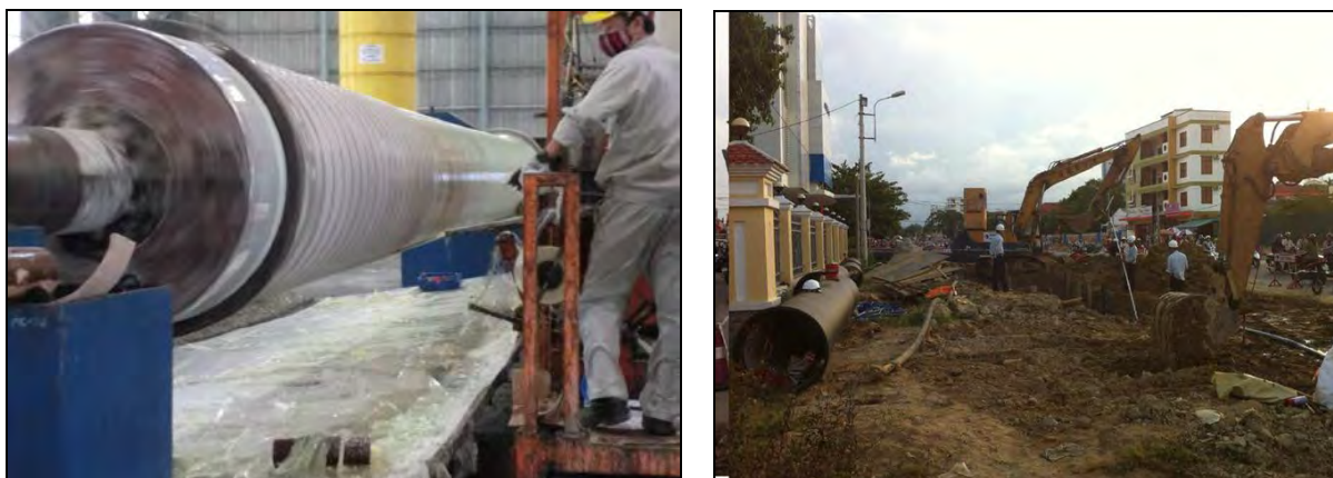
Photo 5.25 (Left) Survey at the Glass-Fiber Reinforced Plastic factory, (Right) Performing of Laying Ductile Iron Pipe
