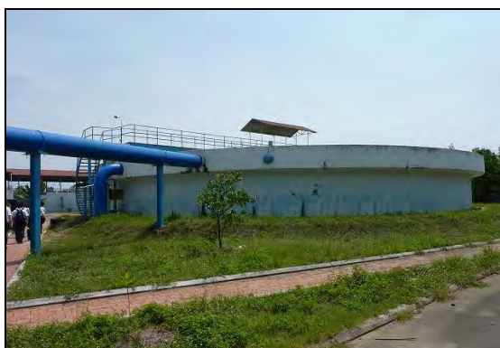
Photo 3.6 Fast Coagulation Basin in San Bay WTP
