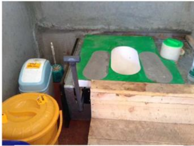
Photo: The Upgraded Squatting GTS Toilets
