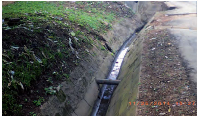
Desilted drainage on a PBC maintained road
