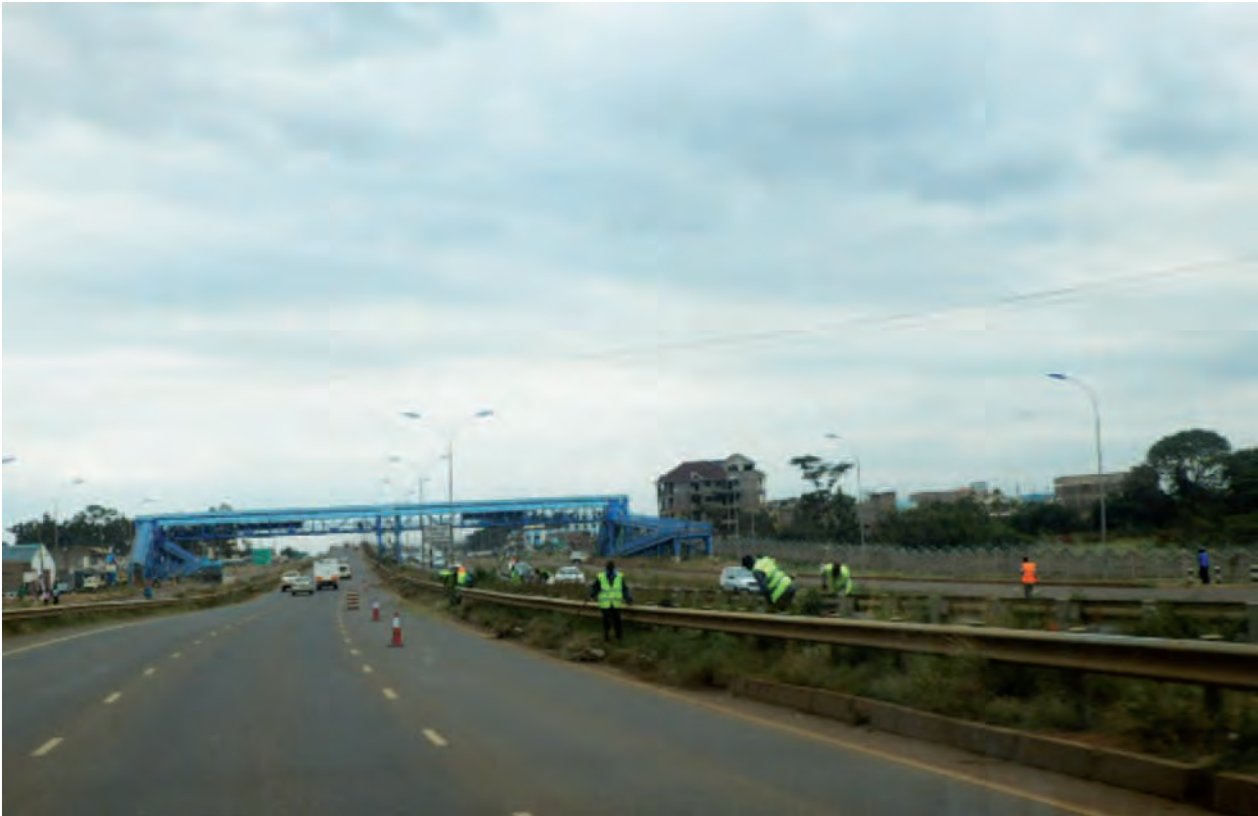
Figure 13-2 Traffic control of Thika Road (grass cutting in the Median)
