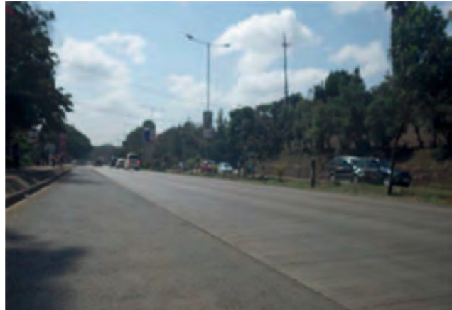
Well maintained carriageway
