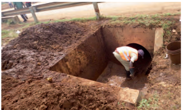
Desilted culvert on a PBC maintained road
