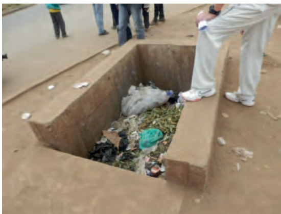
Catch basin full of garbage
