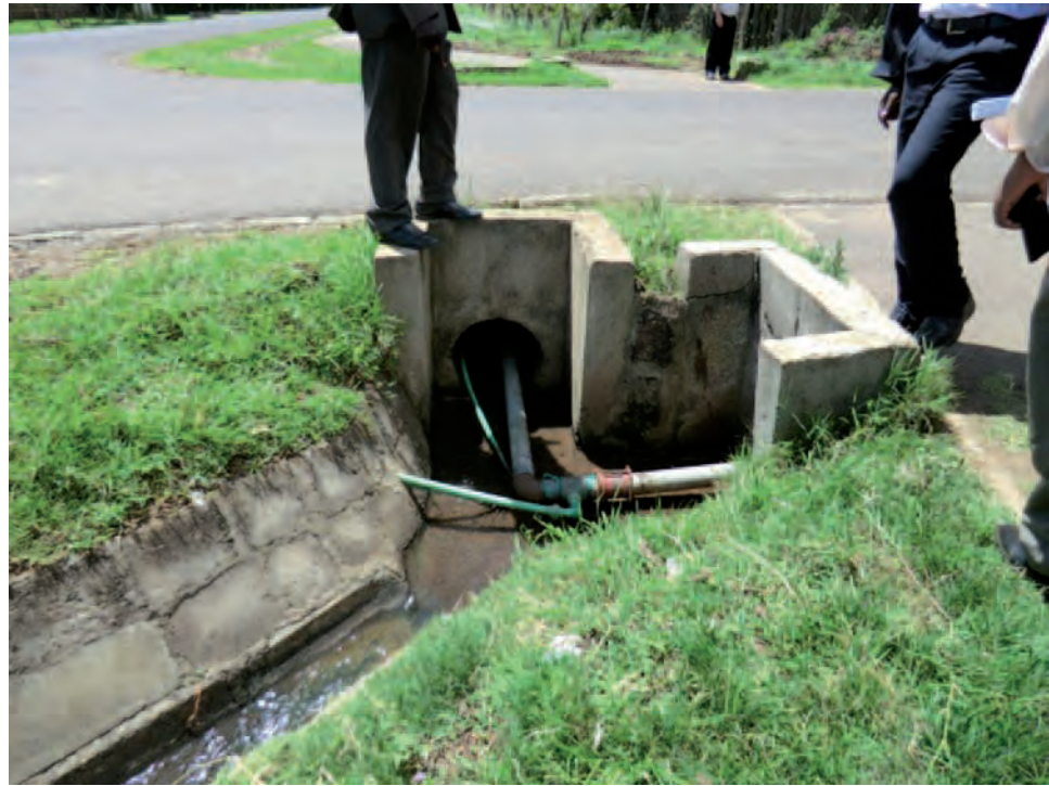
Example : Installation of pipe by private developer
