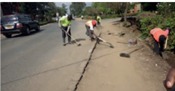
De-siltation of drainage and cleaning of carriageway
