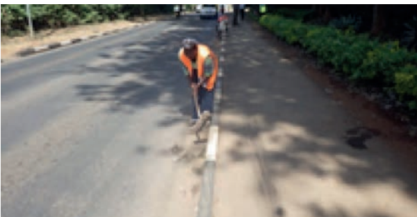
De-siltation of carriageway
