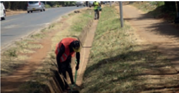
De-silting of drainage
