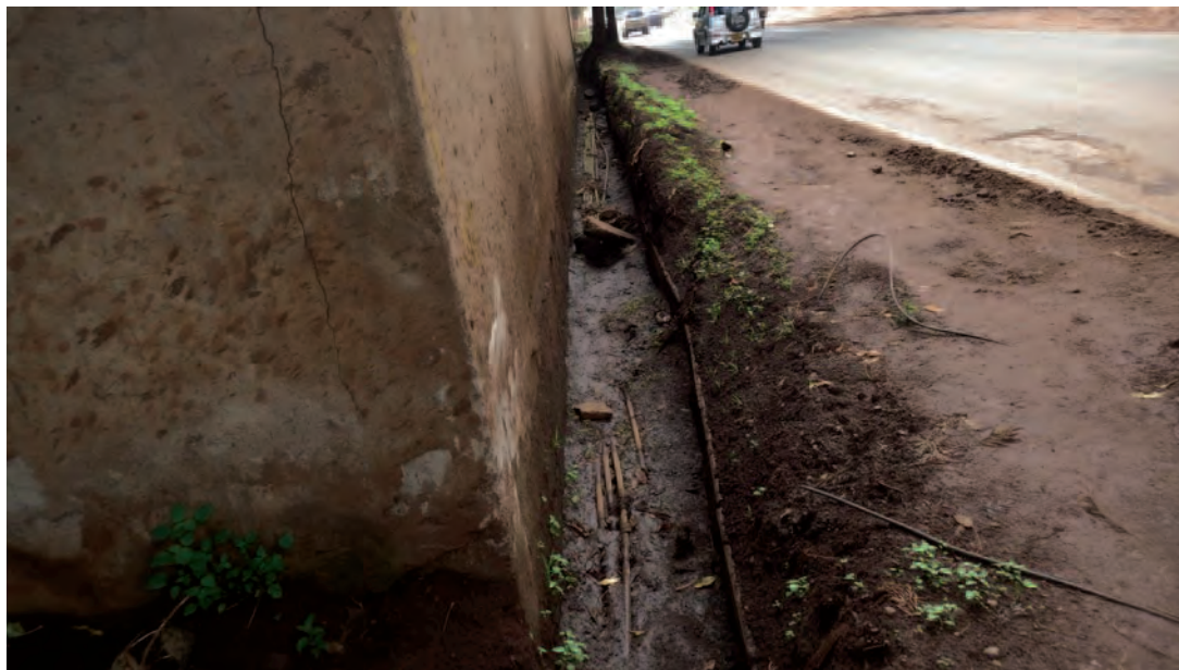
Example: Illegal pipes are found after cleaning the ditch during the Initial Mobilization Period
