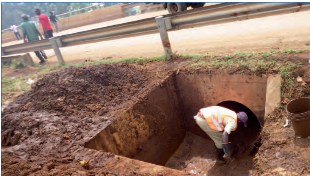
Sample: Clearing culvert to raise service level in Initial Mobilization Period
