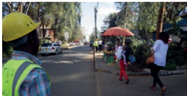
Measurement on de-silted carriageway.
