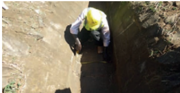
Measurement on De-silted drain
