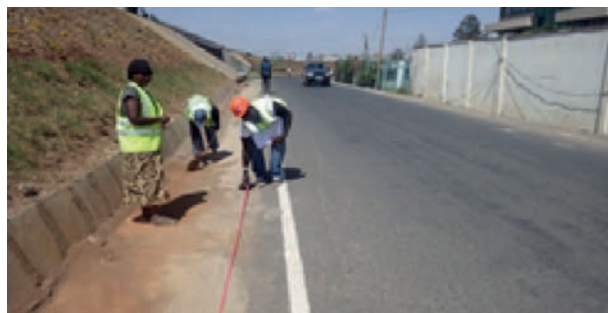
Measurement of completed section
