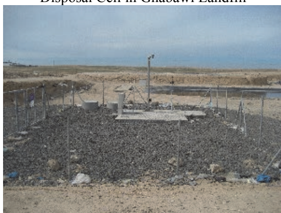
Leachate Circulation System in Ghabawi Landfill
