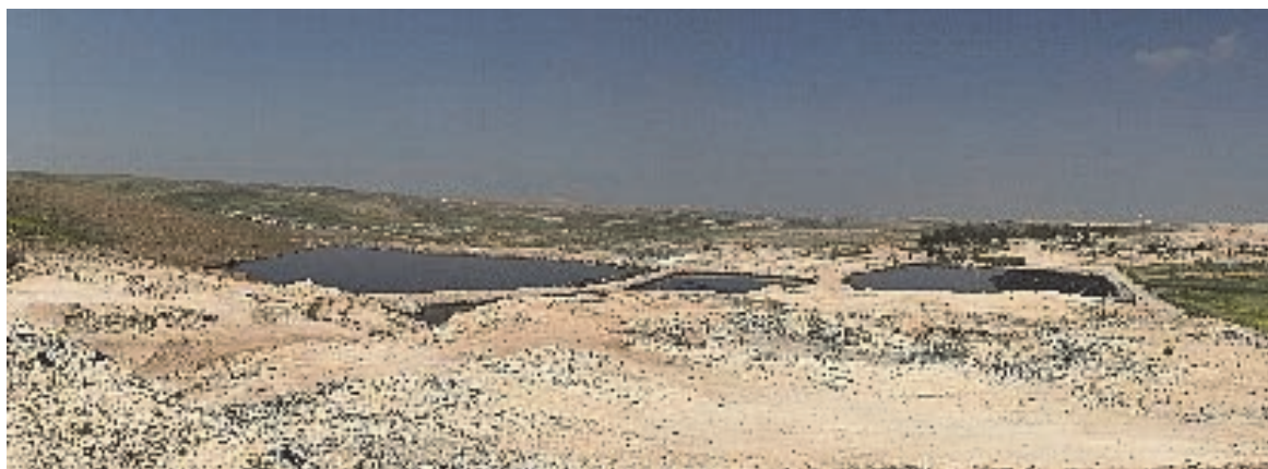
Treatment Pond for Zibar (Wastewater from Olive Oil Factory) in Al Ekaider D/S
