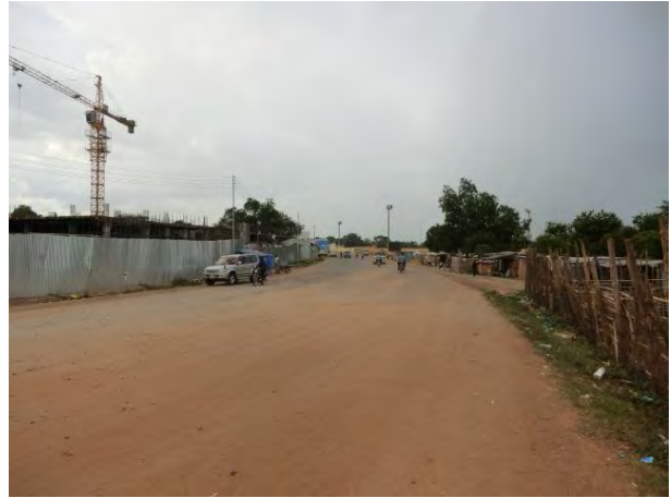
Photo 2-2-3 Current Situation of the Approach Road of Bridge No.7 (Completed until pavement)
