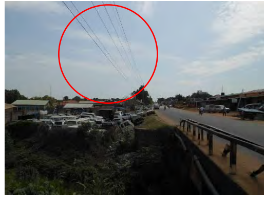
Bridge No.1: Removal of Electric Wire and Pole
