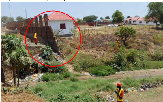
Bridge No.10: Removal of Brick and Masonry Wall
