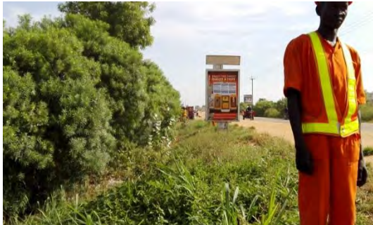
Bridge No.1 Removal of Billboard
