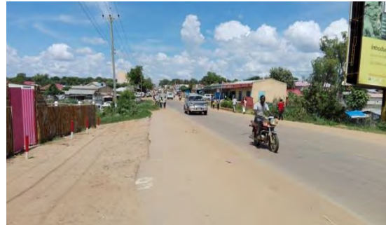
Bridge No.1 Removal of Electric Wire and Pole
