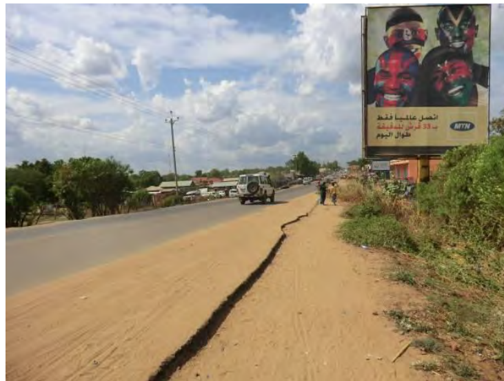
Photo 2-2-1 Current Situation of the Approach Road of Bridge No.1 (Completed until pavement)
