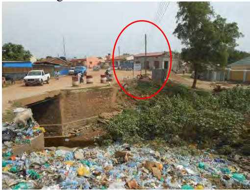
Bridge No.4: Removal of Electric Wire and Pole
