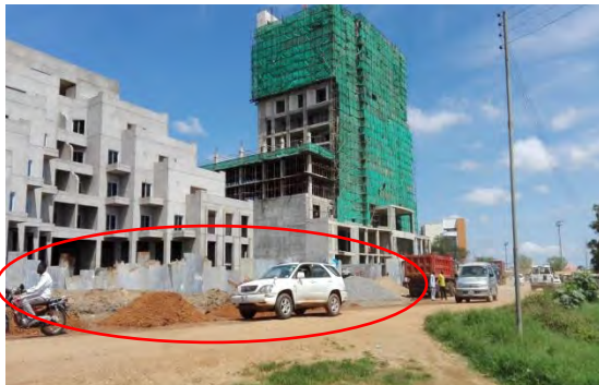
Bridge No.7: Removal of Anseba Hotel Area from Right-of-Way (done)
