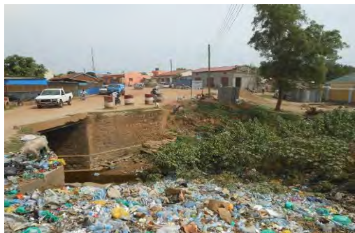
Bridge No.4 Removal of Electric Wire and Pole
