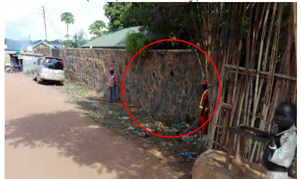
Bridge No.7: Removal of Masonry Wall
