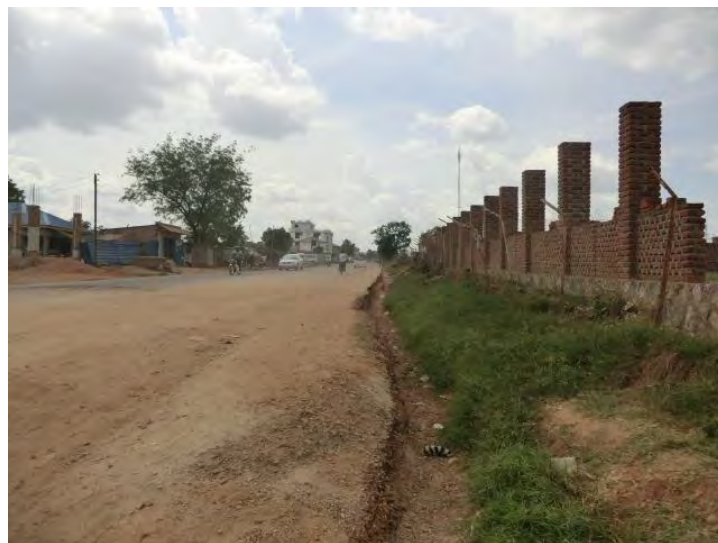
Photo 2-2-4 Current Situation of the Approach Road of Bridge No.10 (Completed until pavement)
