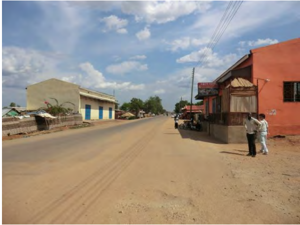
Photo 2-2-2 Current Situation of the Approach Road of Bridge No.4 (Completed until pavement)
