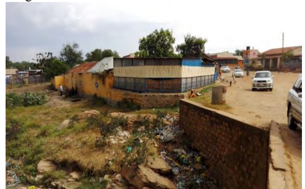
Bridge No.4: Removal of the Part of Existing Restaurant (Now, not necessary)
