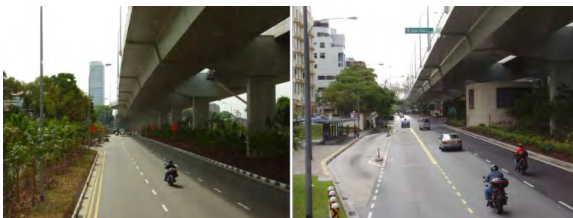
Figure 5.6.3.4 Image of roads in the Thilawa SEZ (Example: The road next to Singapore's container terminal)
