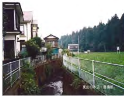
Bank Protection with Concrete Wall
