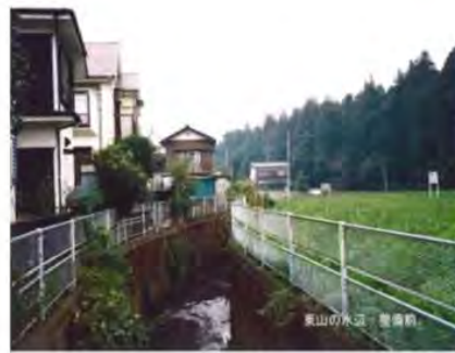
Bank Protection with Concrete Wall
