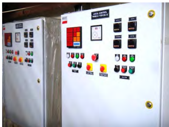
Badra Jassan No. 3 Irrigation Pump Station Installed new control panels
