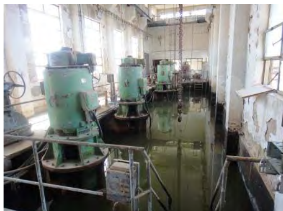
Shakha No. 8 Drainage Pump Station Existing immersed condition (Pump floor)
