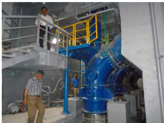
Badra Jassan No. 1 Irrigation Pump Station Installed new pump (front two units)
