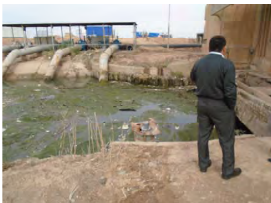
Badra Jassan No. 2 Irrigation Pump Station Existing suction pit diverted by metric pumps
