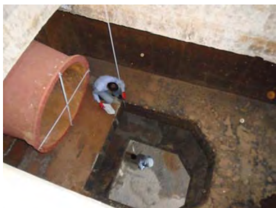
East Gharraf Drainage Pump Station Measurement of existing pump pit
