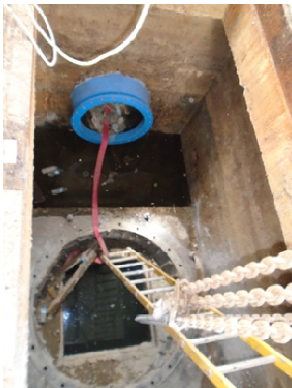
Shakha No. 10 Drainage Pump Station Preparation of base plate for pump
