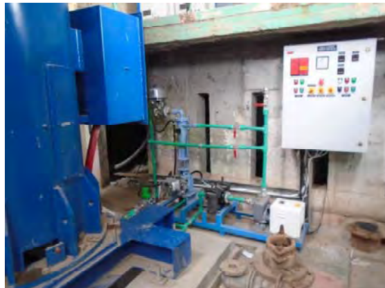
Badra Jassan No. 2 Irrigation Pump Station Installed new pump motor and local switch panel
