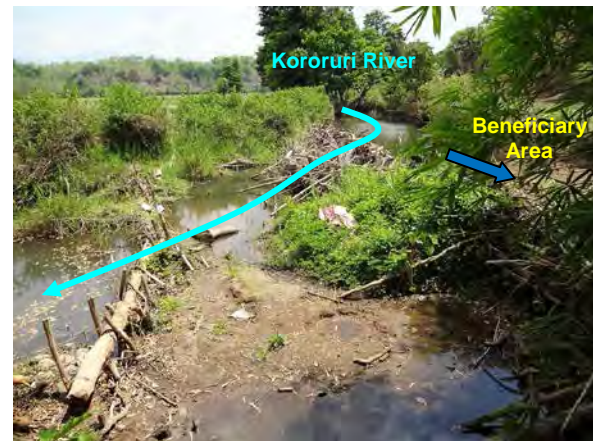
Intake point at Kororuri River
