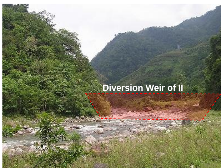
Photo 5-9 Diversion Weir Site of Nyera Amari II
