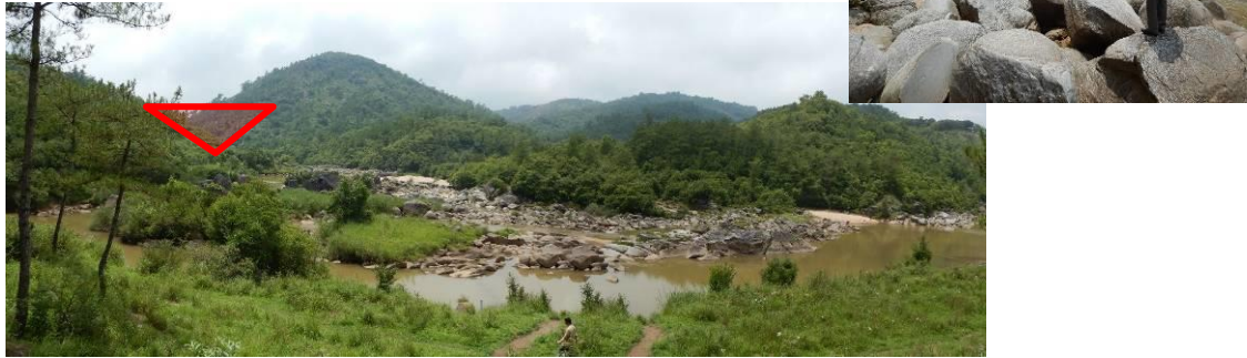
Photo 5-25 Overview of the Dam Site (Umngi Storage Site)
