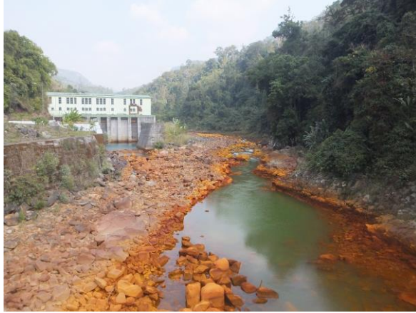
Photo 5-22 Rock Condition along the riverbed downstream of the Myntdu Leshka I powerhouse
