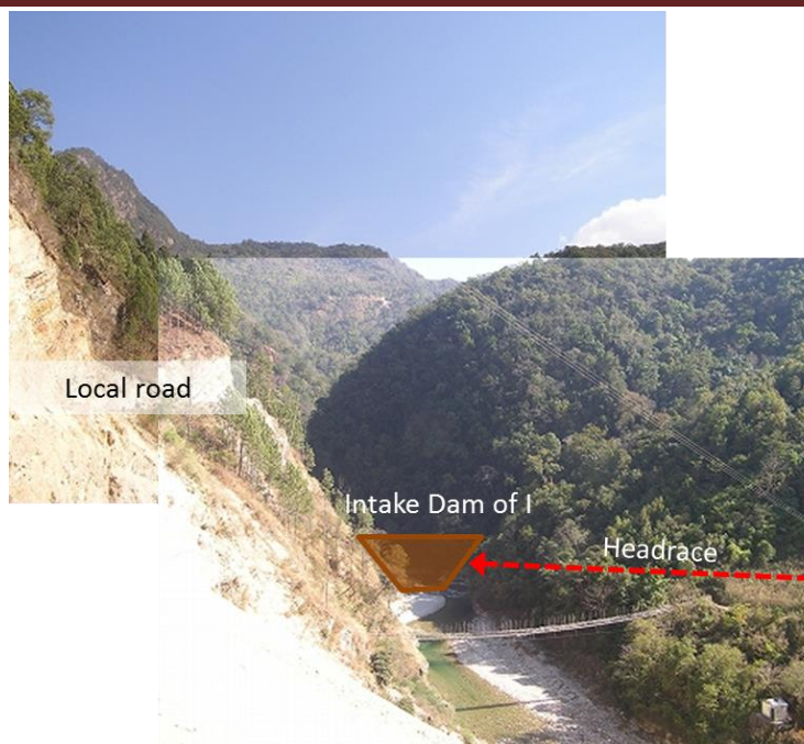
Photo 5-8 Intake Dam Site of Nyera Amari I
