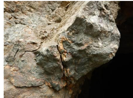
Photo 5-16 The rock at the left bank of the dam site
