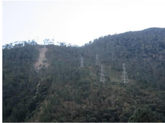
400kV T/L Under Construction
