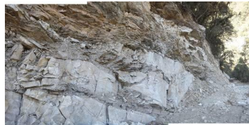
Photo 5-19 The rock on a cutting Slope
