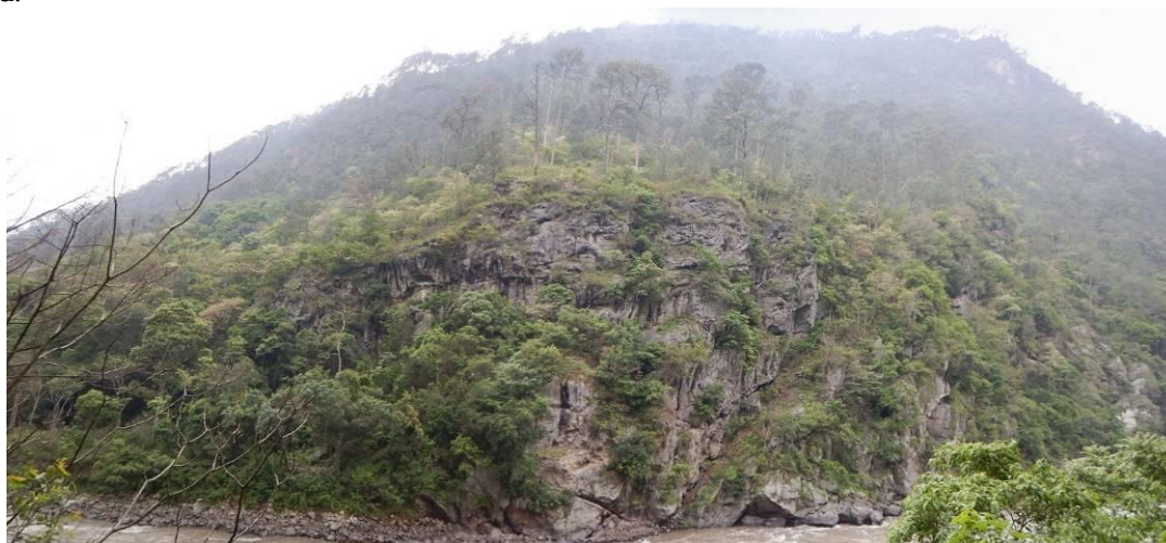
Photo 5-15 Overview of right bank of dam, where intake is also planned
