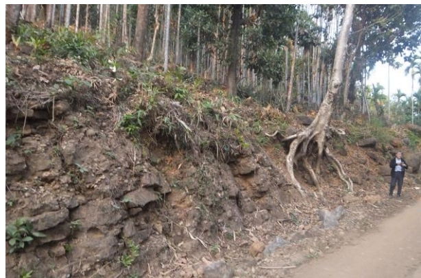
Photo 5-24 Hard and Fresh Granite in the backyard of the Myntdu Leshka I powerhouse
