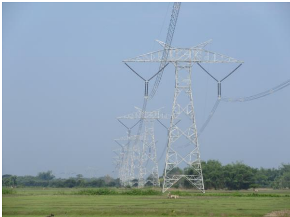
±800kVDC T/L Under Construction
