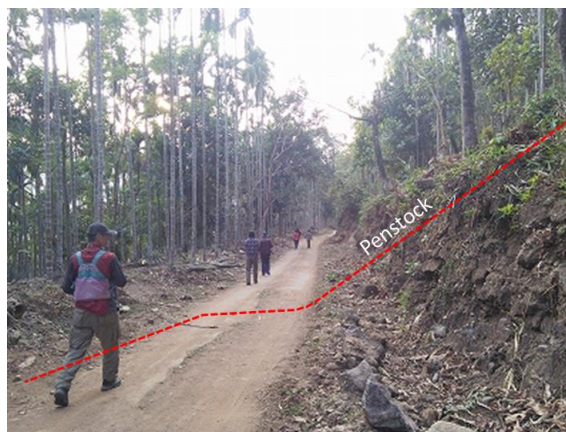
Photo 5-13 Power House Site of Myntdu Leshka II
