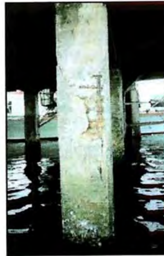
Badly damaged concrete pile of deck
