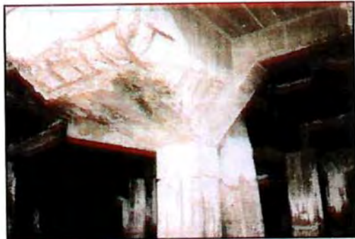
Peeled concrete cover and exposed re-bars
