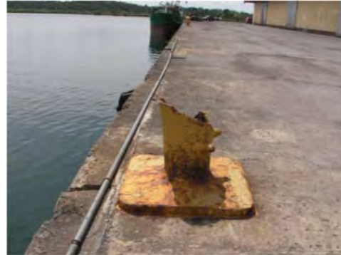
Photo: Damaged Bollards
