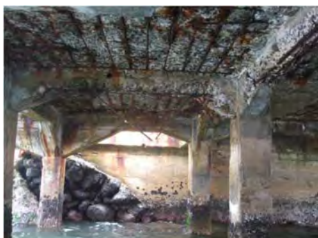
Photo of superstructure
