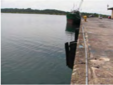
Photo: Damaged Fenders
