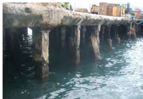
Photo of piles
