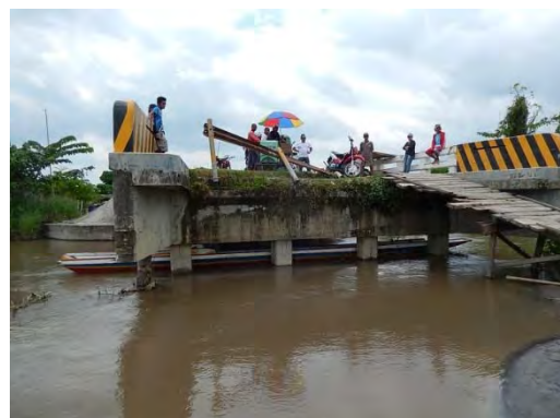
Destroyed Pan-Philippine Highway near Lambayong by course change on Ala River (September 7, 2015)
