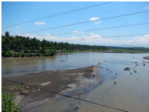
Simuay River upstream of bridge on Pan-Philippine Highway (May 30, 2015)
