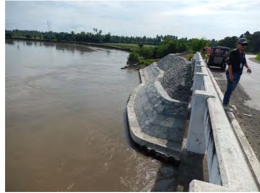
Tentative protection work of left abutment of Tunggol Bridge (September 7, 2015)
