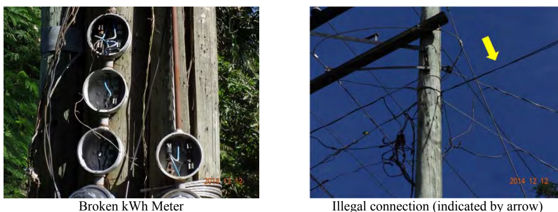
Figure 3.4 kWh Meters Installed in Franchise Area of MAGELCO
