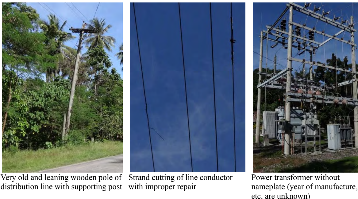
Figure 3.2 Distribution Line Facilities of MAGELCO
