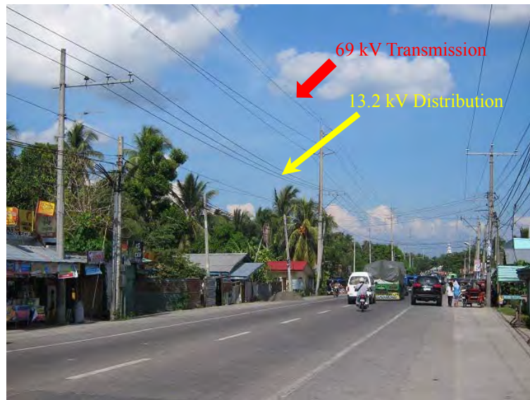
Figure 1.13 Transmission and Distribution Lines in Cotabato City
