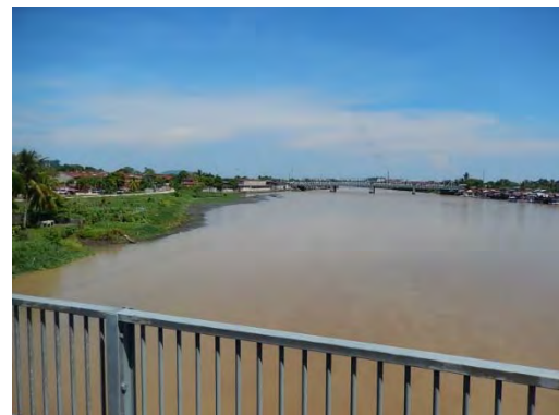
Rio Grande de Mindanao downstream of Delta Bridge (May 30, 2015)
