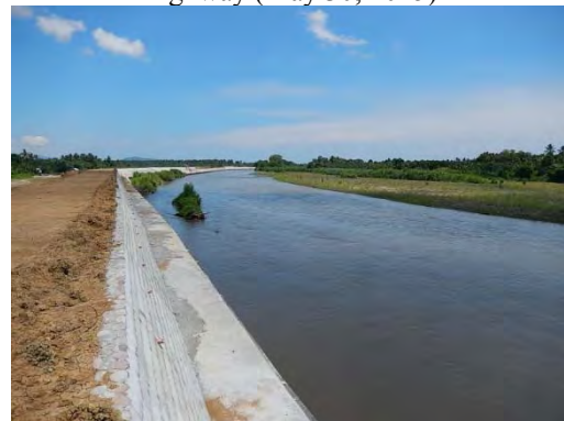
Newly constructed closing dike on left bank of Simuay River (May 30, 2015)
