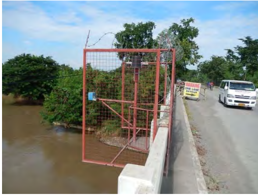
Telemetered water-level and rainfall censors of Project NOAH on Tunggol Bridge (September 7, 2015)
